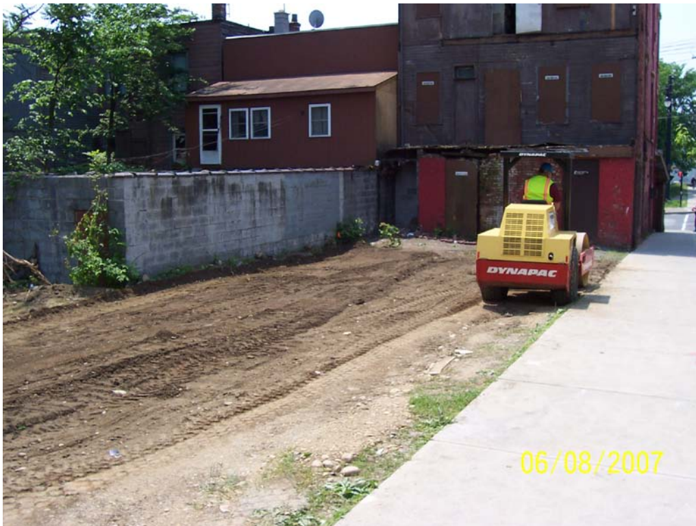
PHOTO 22. Southerly view of final backfilling and grading at SRA-2.
