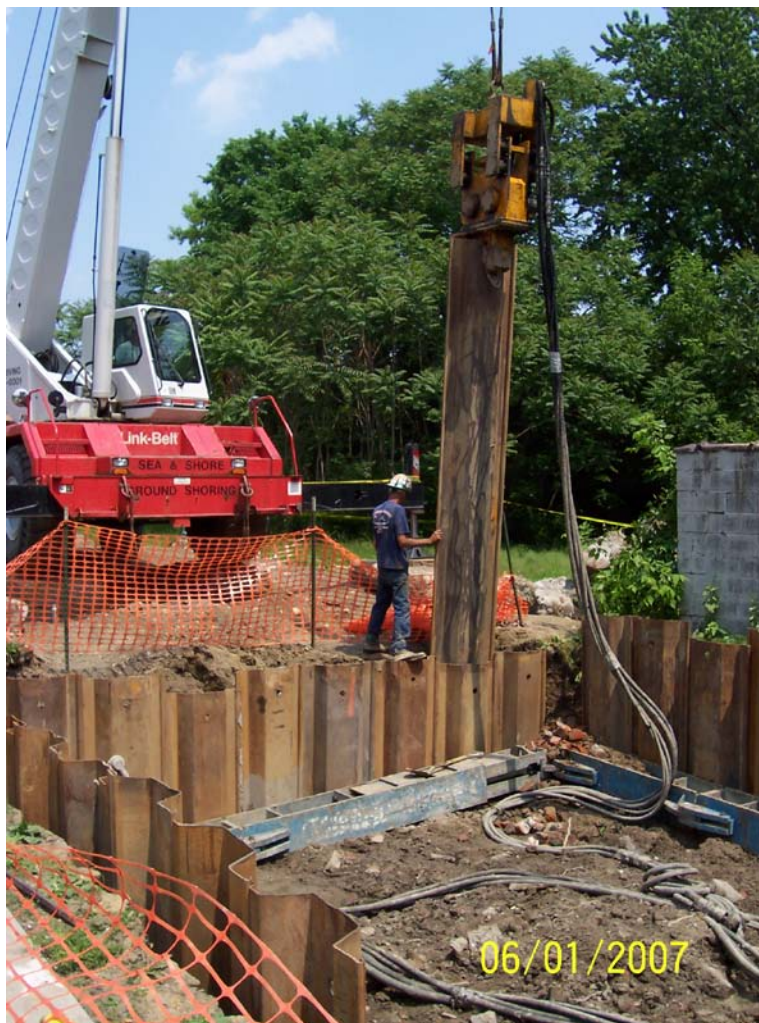
PHOTO 13. Northeasterly view of sheeting placement at SRA-2.
