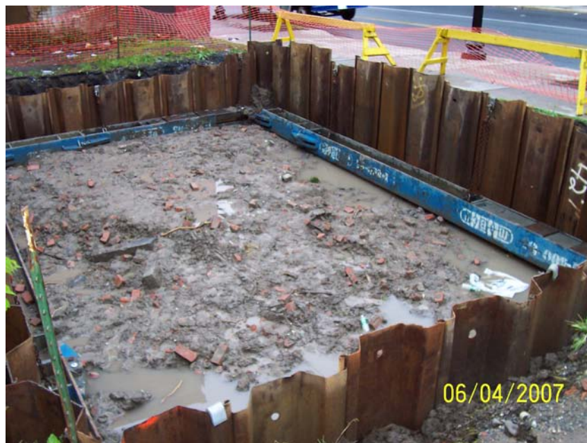
PHOTO 14. Southwesterly view of sheeting at SRA-2.
