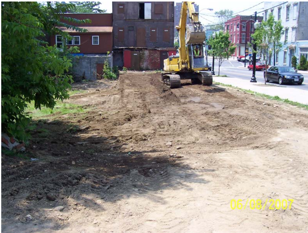
PHOTO 21. Southerly view of final backfilling and grading at SRA-2.
