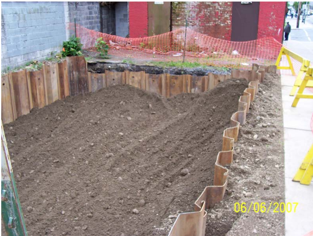
PHOTO 19. Southerly view of backfilling at SRA-2.
