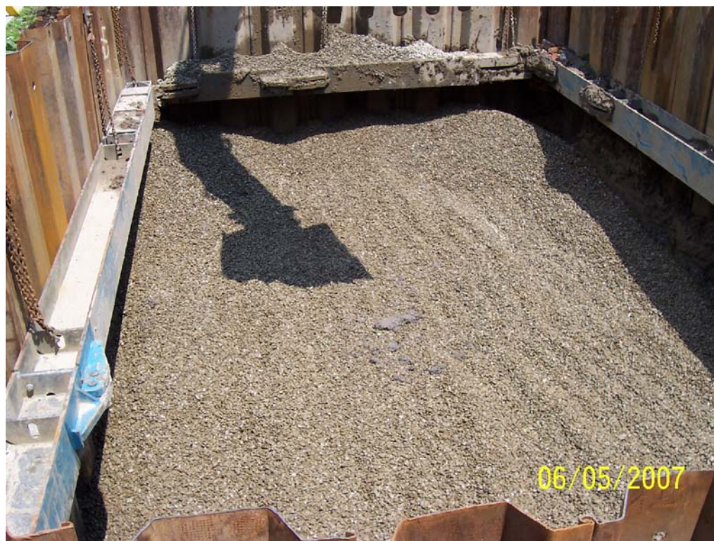
PHOTO 18. Northeasterly view of stone backfill at SRA-2.
