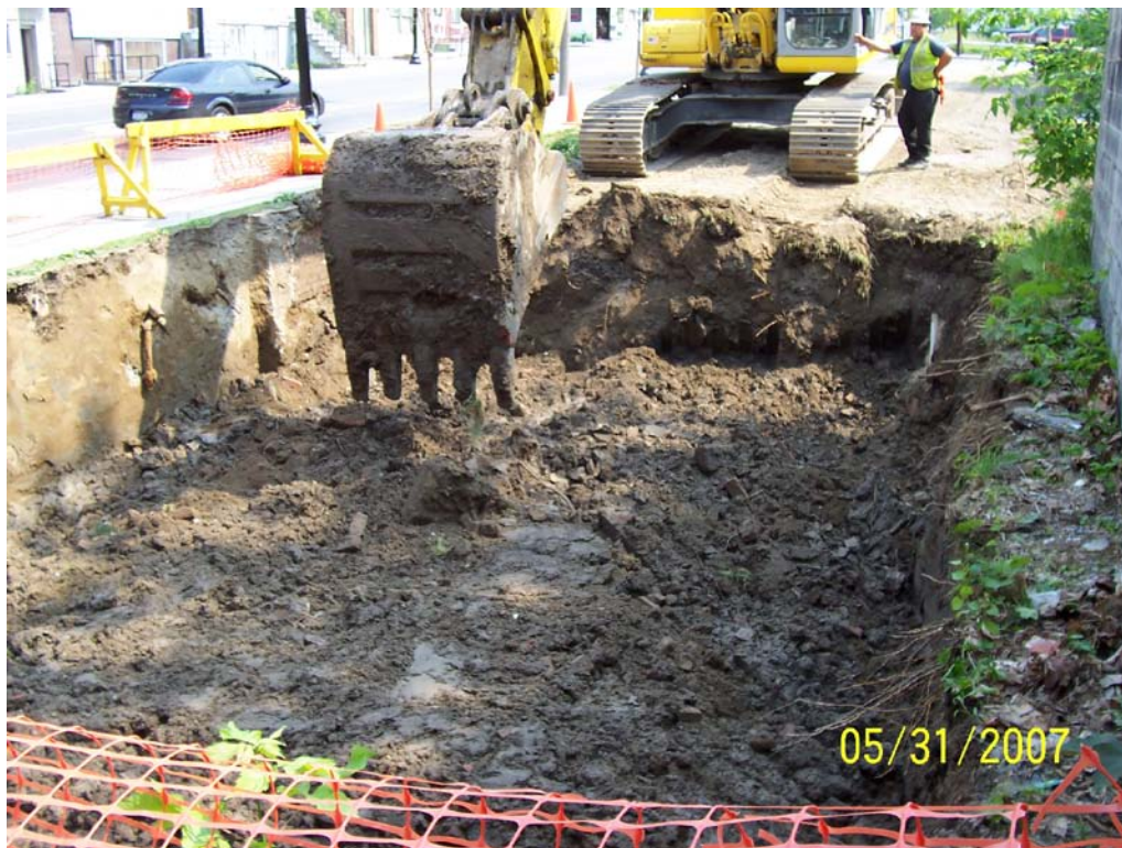
PHOTO 12. Northerly view of SRA-2 prior to sheeting placement.
