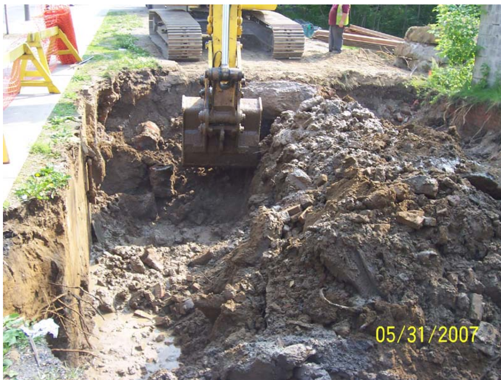
PHOTO 10. Northerly view of removal of concrete foundation at SRA-2.
