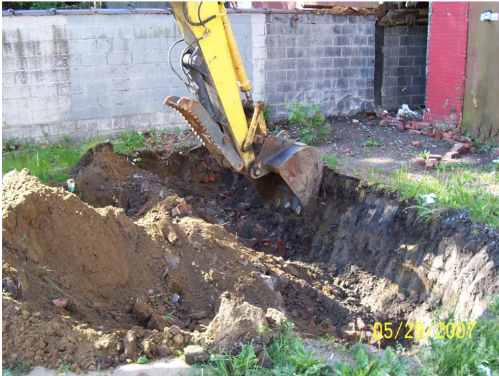
PHOTO 7. Southeasterly view of SRA-2.
