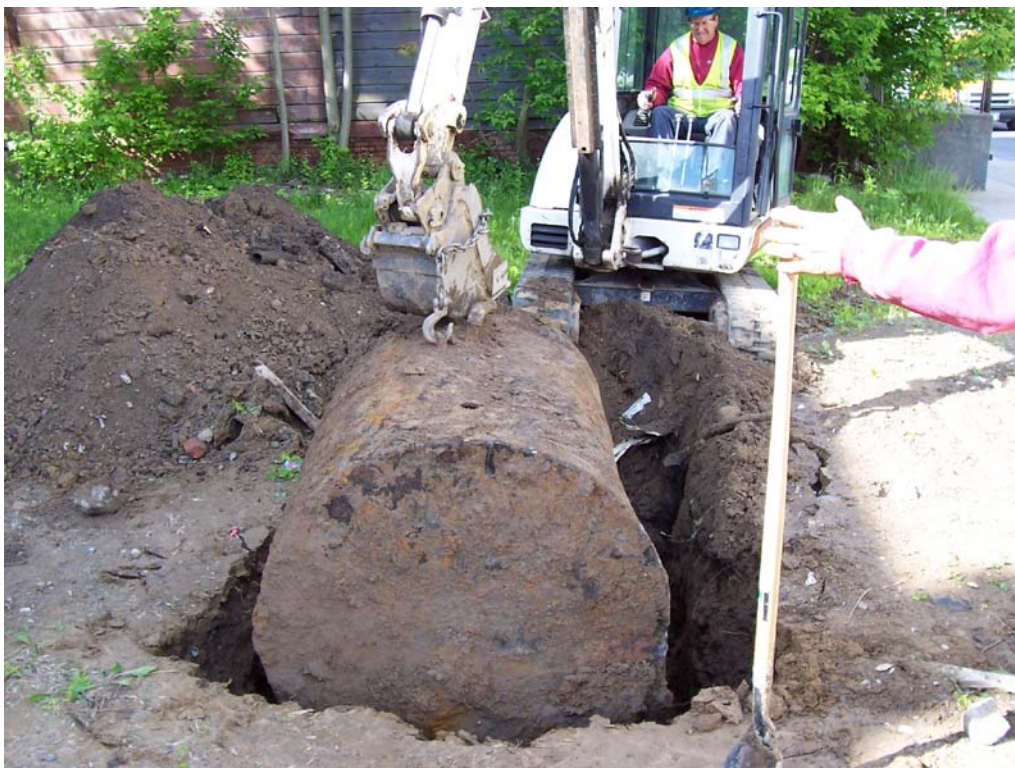
PHOTO 2. Southerly view of UST removal at SRA-1.
