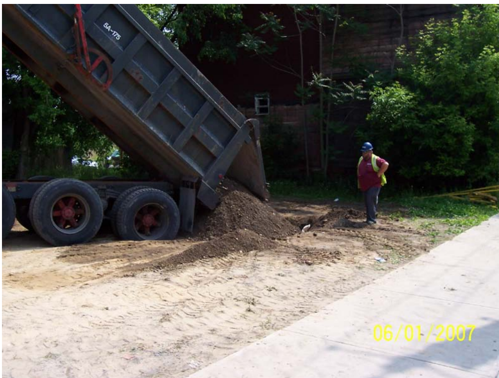
PHOTO 6. Southeasterly view of backfilling at SRA-1.
