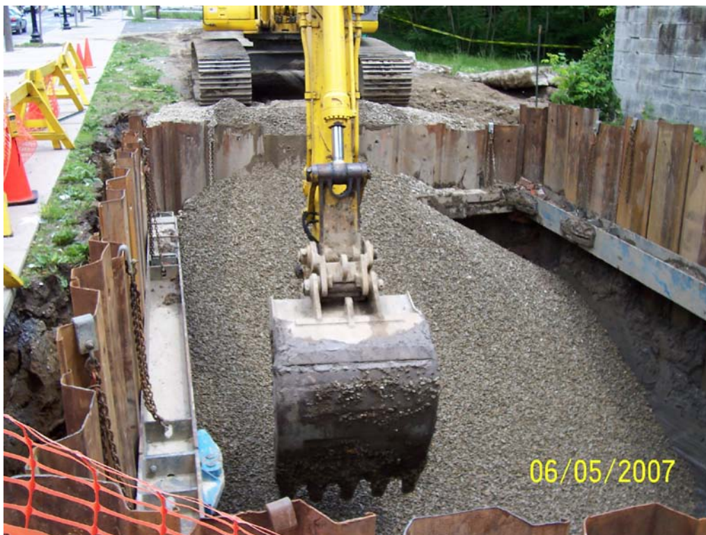
PHOTO 17. Northeasterly view placing stone backfill at SRA-2.
