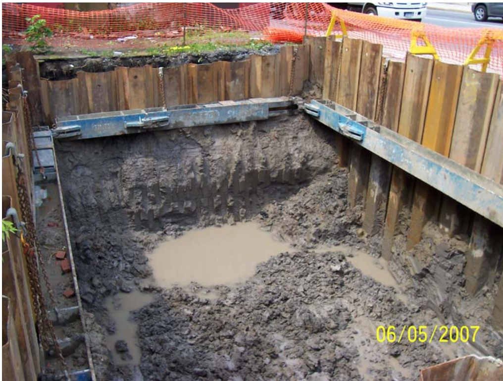
PHOTO 15. Southwesterly view of SRA-2 excavation within sheeting.
