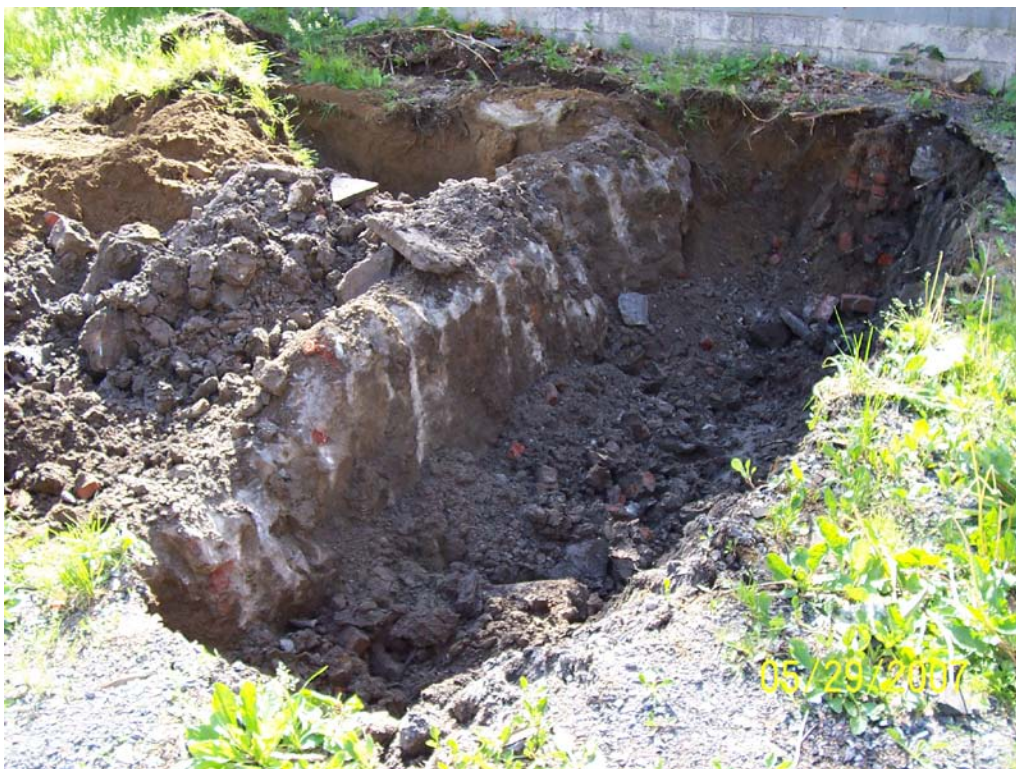
PHOTO 8. Northeasterly view of concrete foundation at SRA-2.
