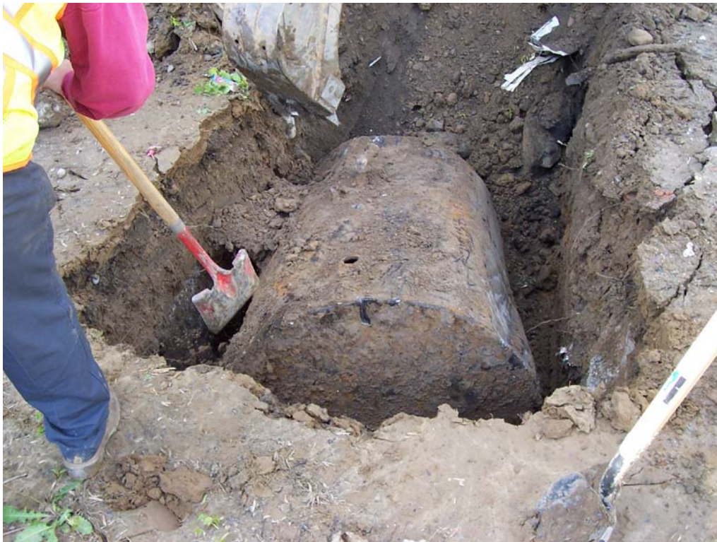
PHOTO 1. Southerly view of UST at SRA-1.
