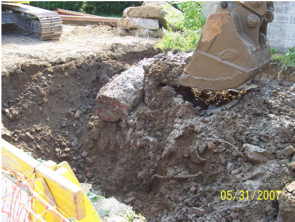
PHOTO 11. Northeasterly view of removal of concrete foundation at SRA-2.
