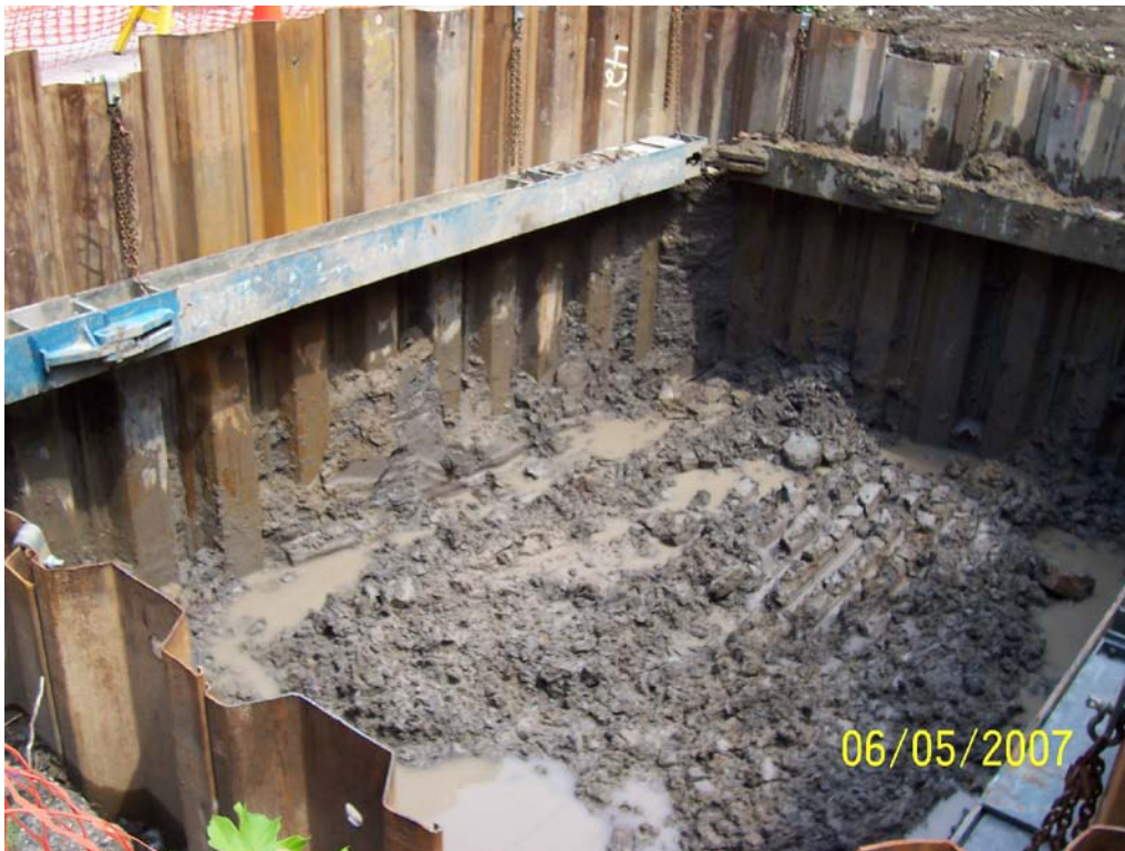
PHOTO 16. Southeasterly view of maximum excavation depth within sheeting at SRA-2.
