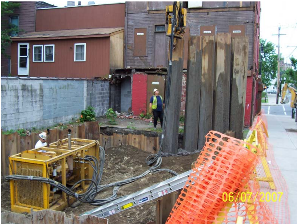
PHOTO 20. Southerly view of sheeting removal at SRA-2.
