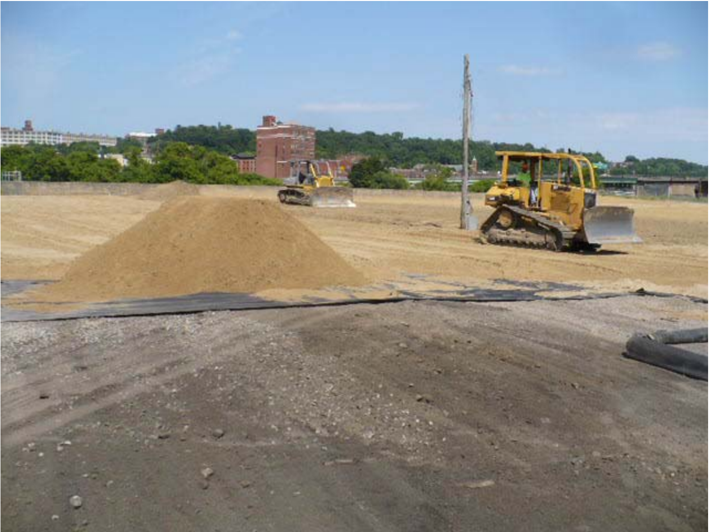
Placement of soil cover on graded site
