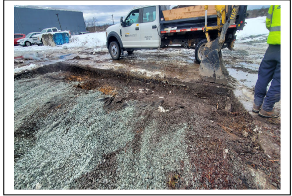
Breach area cleared down to existing fabric.
