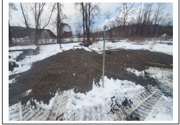
12" of No. 2 Stone placed over fabric in flywheel area.
