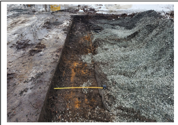
Breach area fabric cut away to prepare overlap of new fabric.
