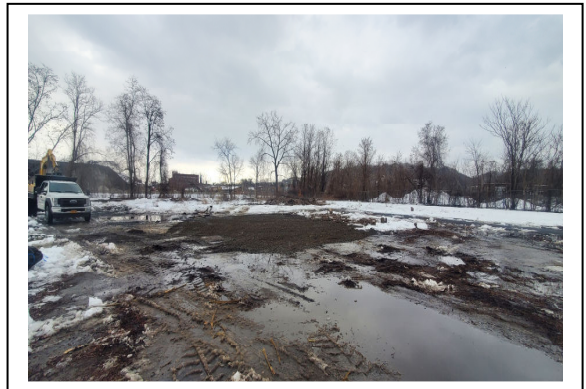
Completed repair of breach with 12" of No. 2 Stone over fabric.
