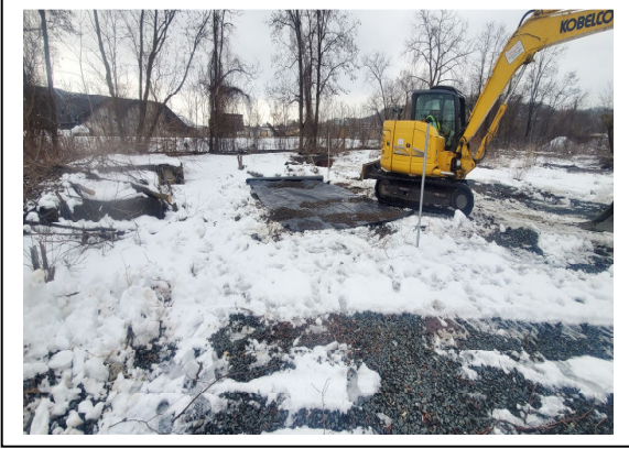
Fabric being spread over flywheel area looking north.
