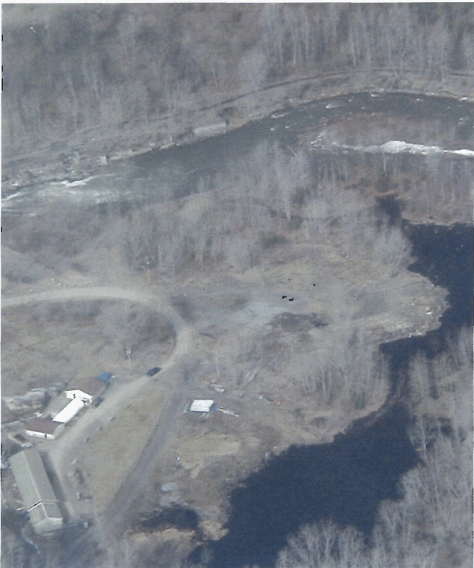
Town Waste Water Treatment Plant with Black Ash Pond in foreground
