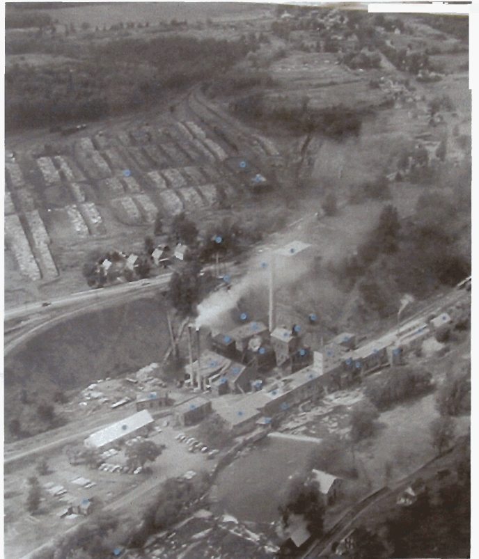
Former Pulp Mill
