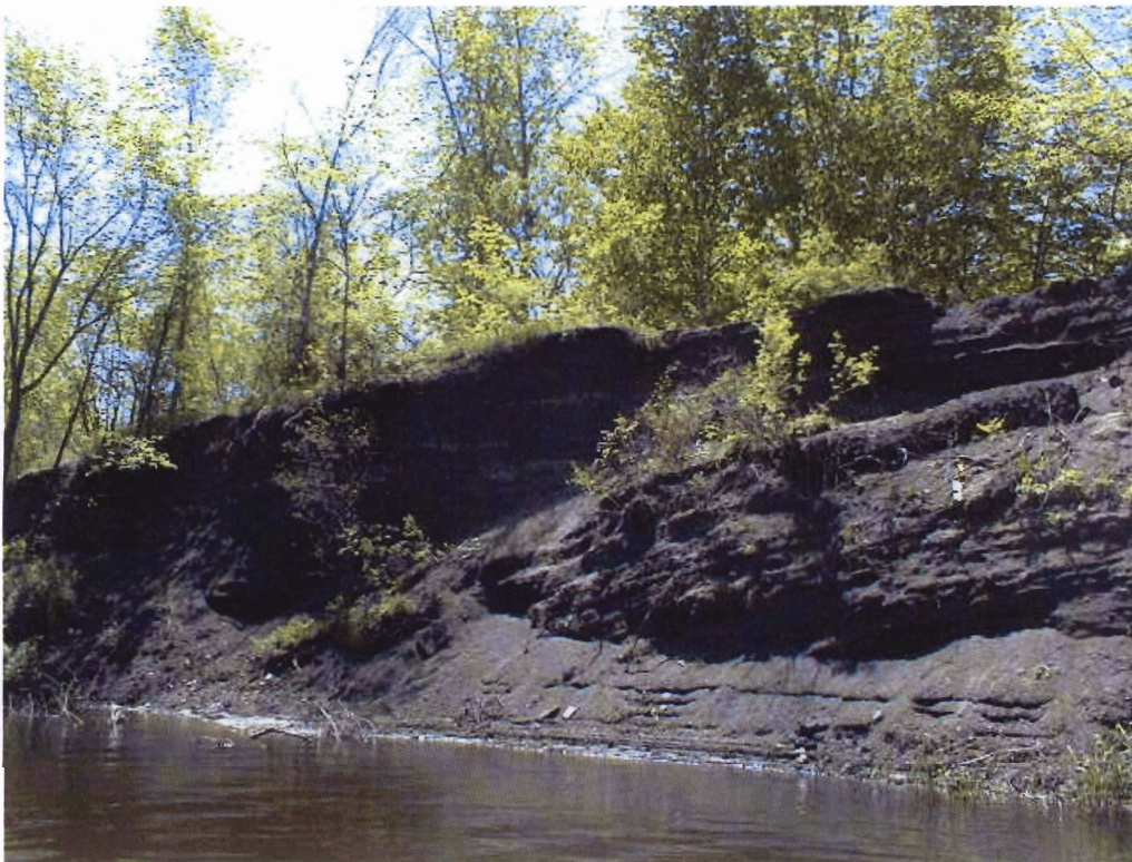
Black ash collapsing into the river
