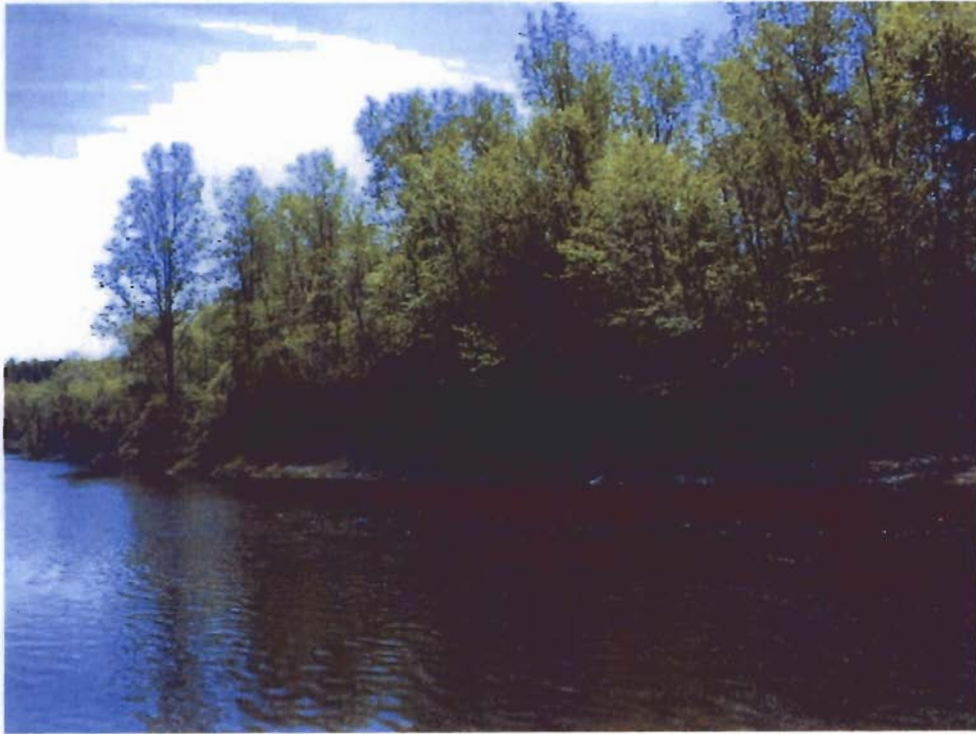
View from the river of the eroded bank
