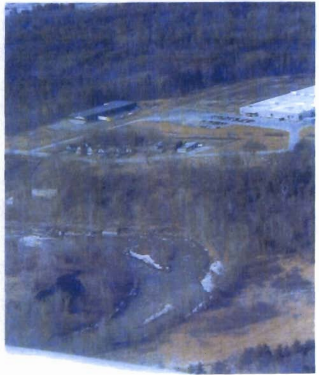
Black Ash Pond and Sludge Lagoon, looking west
