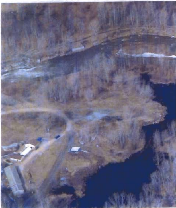
Town Waste Water Treatment Plant with Black Ash Pond in foreground
