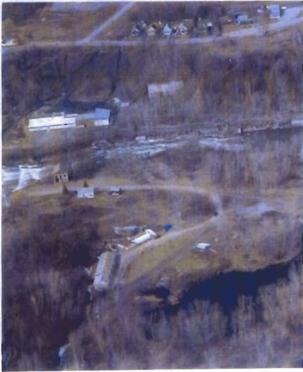
Black Ash Pond, looking west
