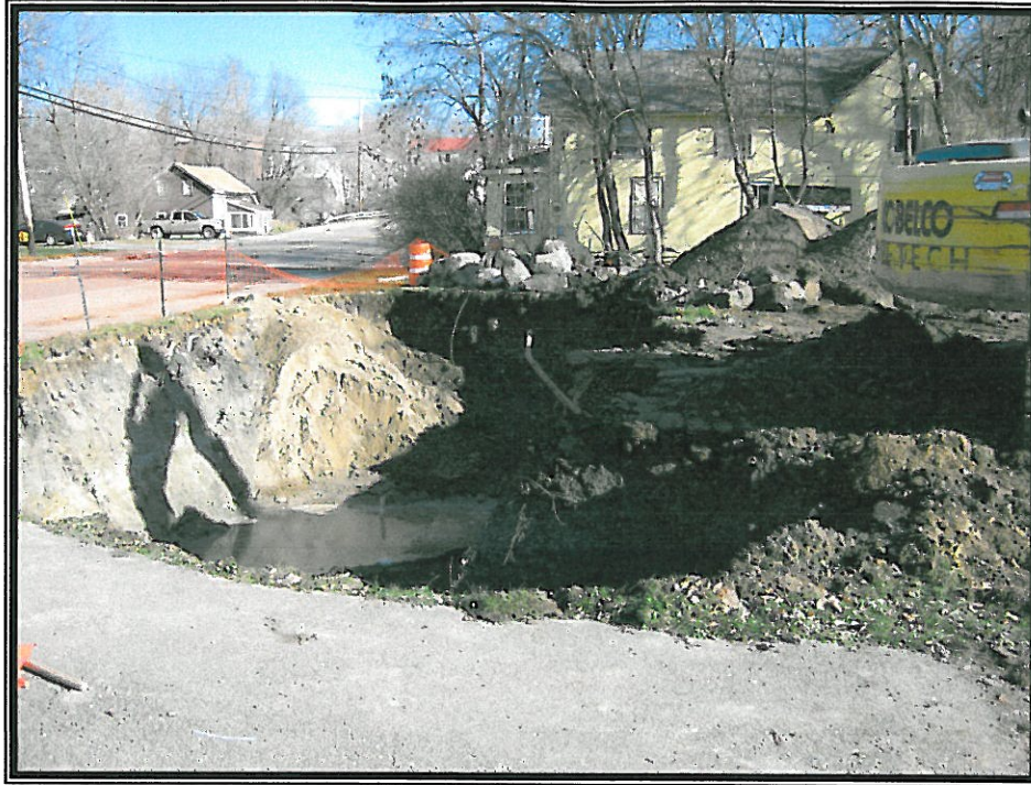
Photograph 1: Northern Excavation Wall and Progressing Excavation Area
