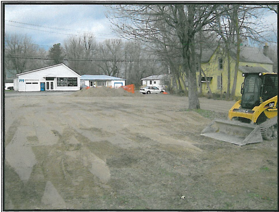
Photograph 4: Subject Property Backfilled and Graded.
