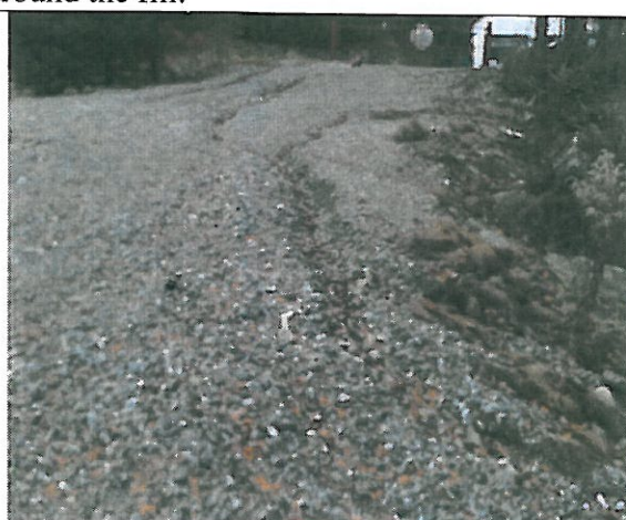
Stromwater runoff from Old Lake Colby Drive is running down the access road and beginning to erode the access road. The Village is currently looking at options for ensuring that stormwater from the road does not enter the site.
