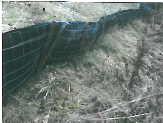
The silt fence is in good condition in most areas around the fill.
