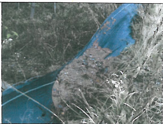
The silt fence was breached in one location. This issues was corrected in May 2014.
