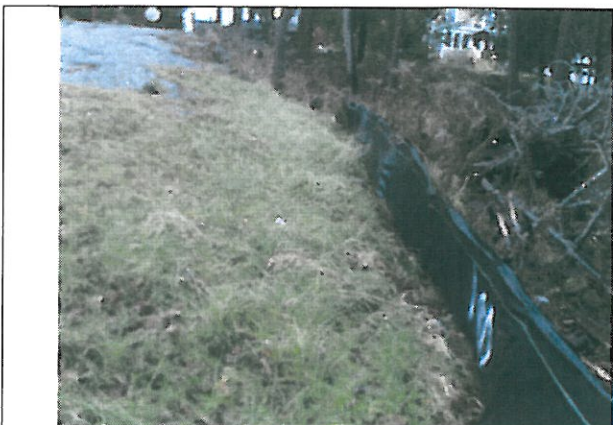
Side Slopes of the fill on the southern and western property boundaries have be fairly well stabilized
