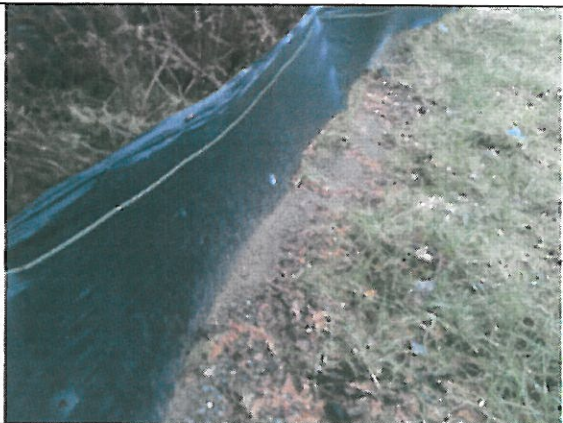
There is some movement of sediment from the fill site, but the silt fence is doing a good job in trapping the sediment so that it does not leave the site.
