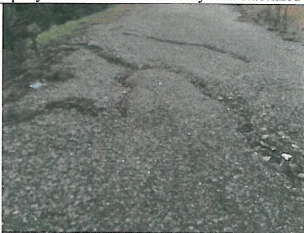
Stromwater runoff from Old Lake Colby Drive is running down the access road and beginning to erode the access road. The Village is currently looking at options for ensuring that stormwater from the road does not enter the site.
