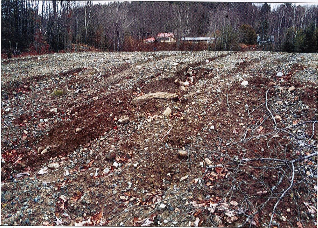
Gully erosion on the western side of the site. This area was stabilized after the November 6, 2015 inspection. A current picture of this site is provided below.
