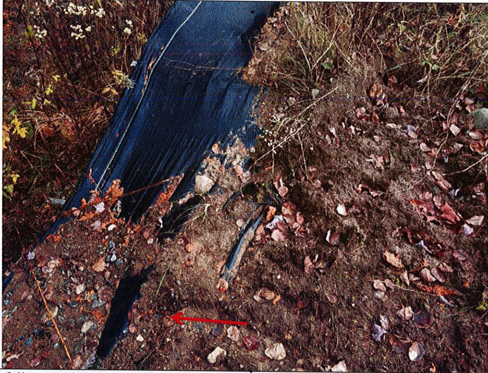
Silt fence failure (11/6/2015). All silt fences were repaired/replaced during the middle of November 2016.
