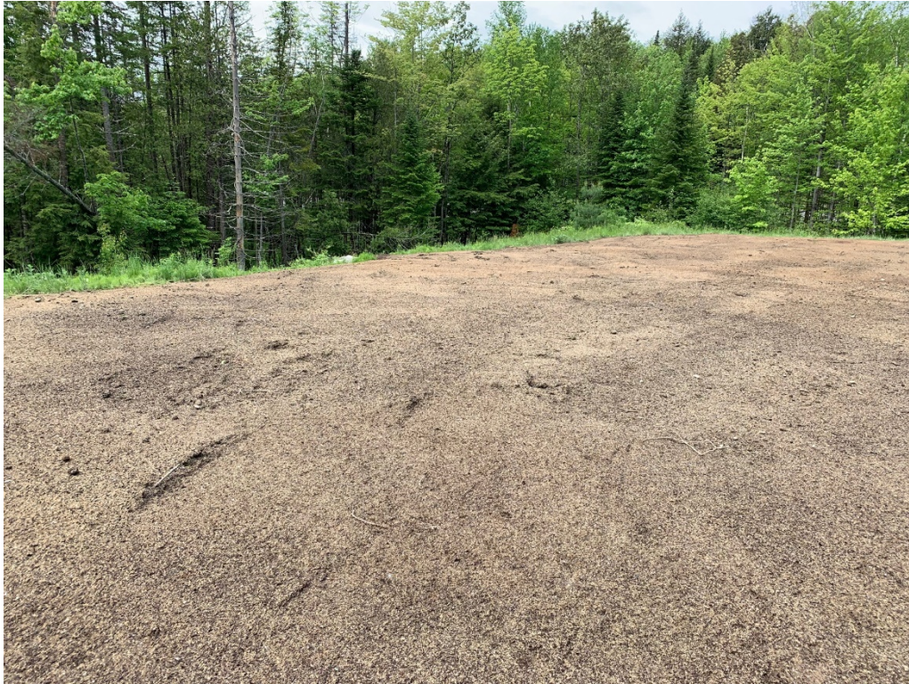
Figure 1 View of completed cover with topsoil and hydroseed
