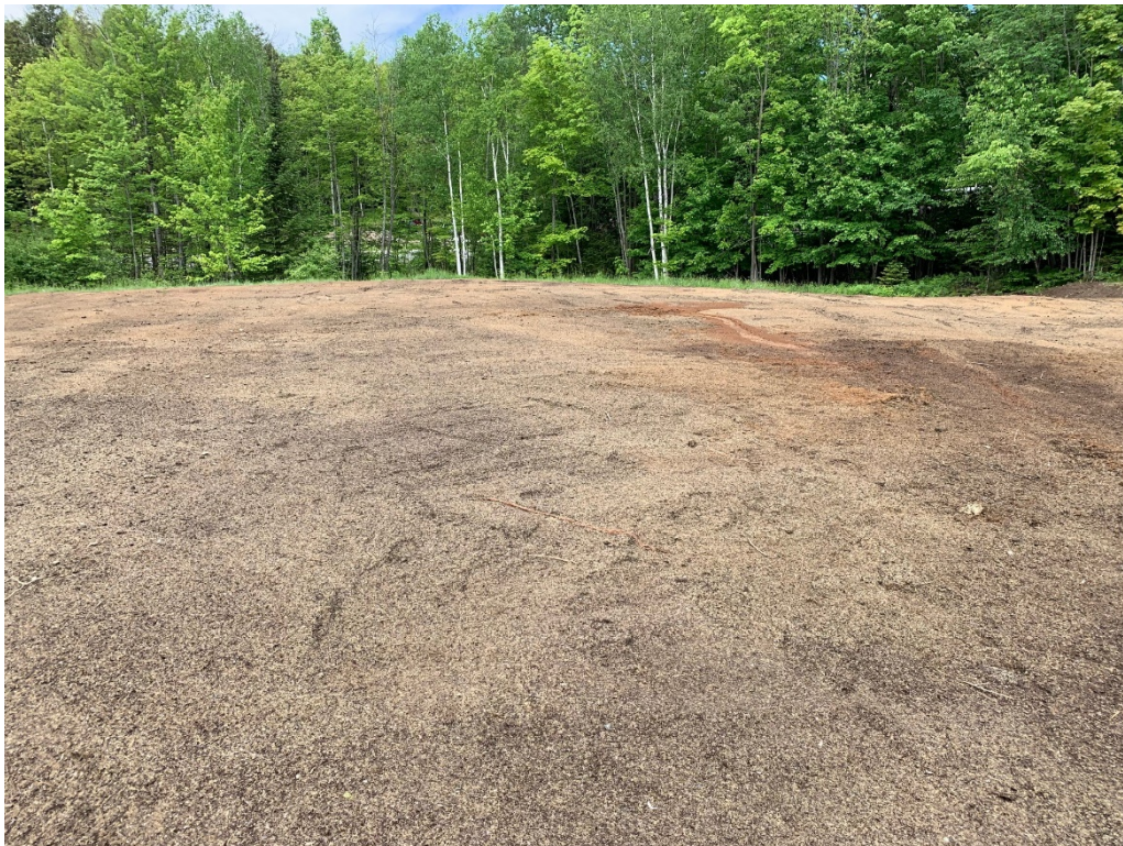
Figure 2 View of completed cover with topsoil and hydroseed
