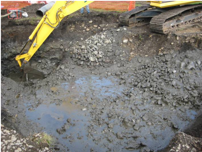
Excavation of Cobbles (around 6-8' below ground surface) and Groundwater/Soil Slurry - September 10, 2008
