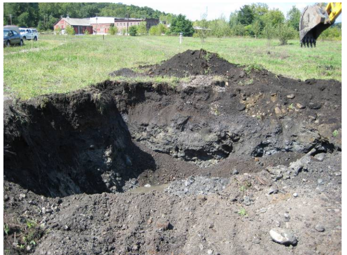
Excavation of Contaminated Soils September 8, 2008
