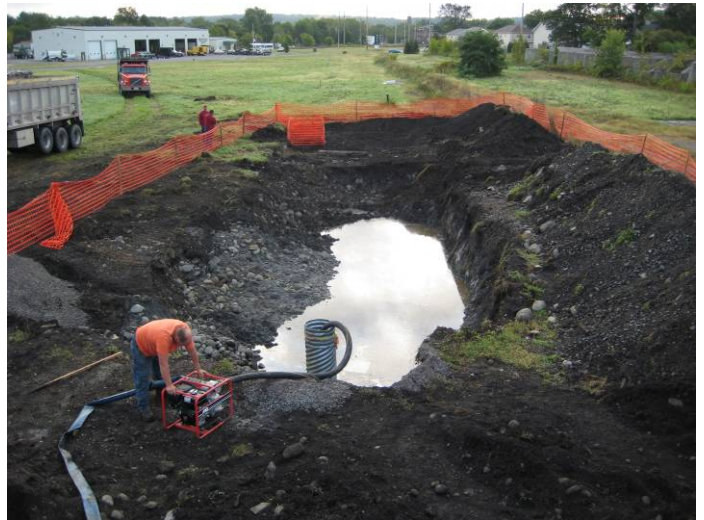
Excavation and dewatering system, security fencing visible, Camera facing northeast - September 11, 2008
