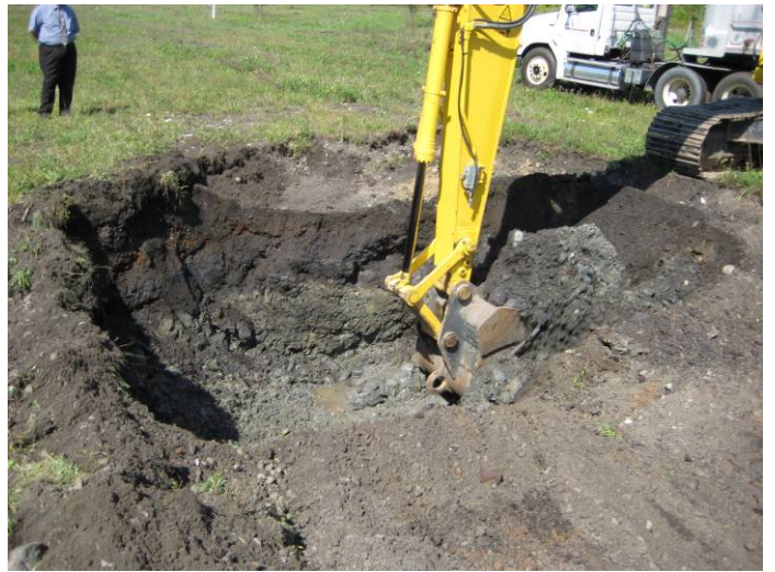
Excavation of Contaminated Soils September 8, 2008
