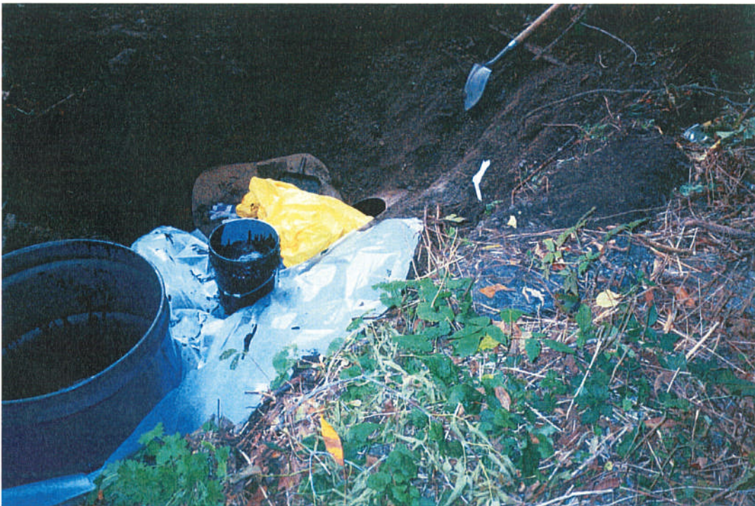
Top: Uncovering first UST
