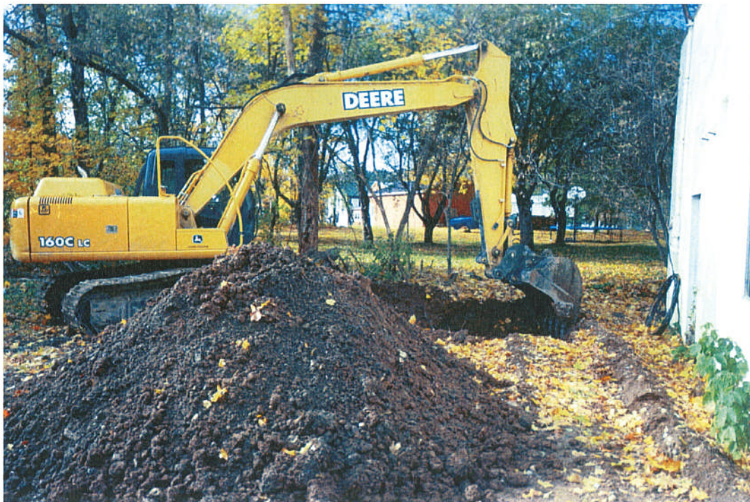
Top: View looking west at the beginning of November 3, 2005 Soil Removal Bottom: Removal of backfill placed October 5, 2005
