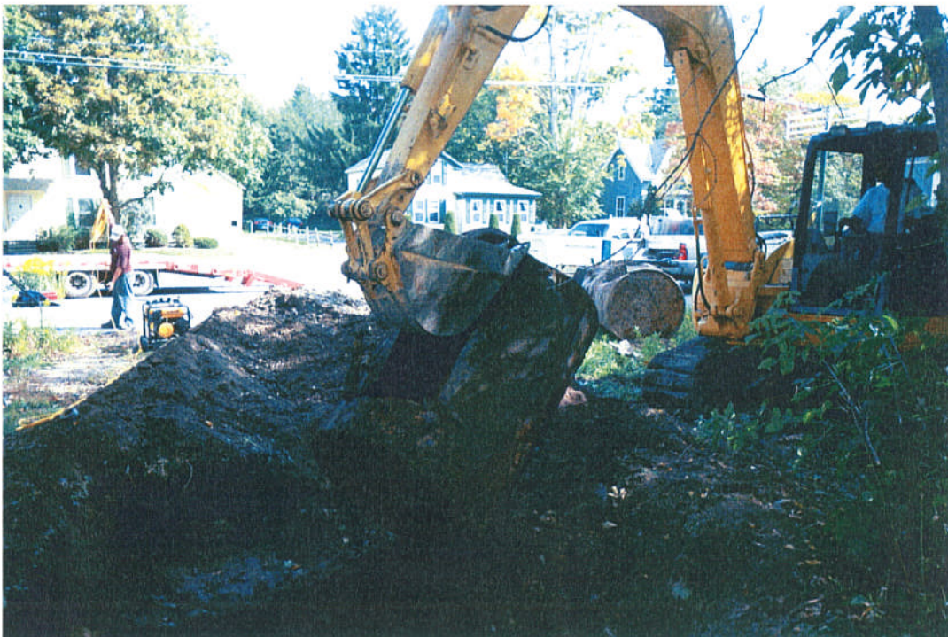
Top: Uncovering top of second UST
