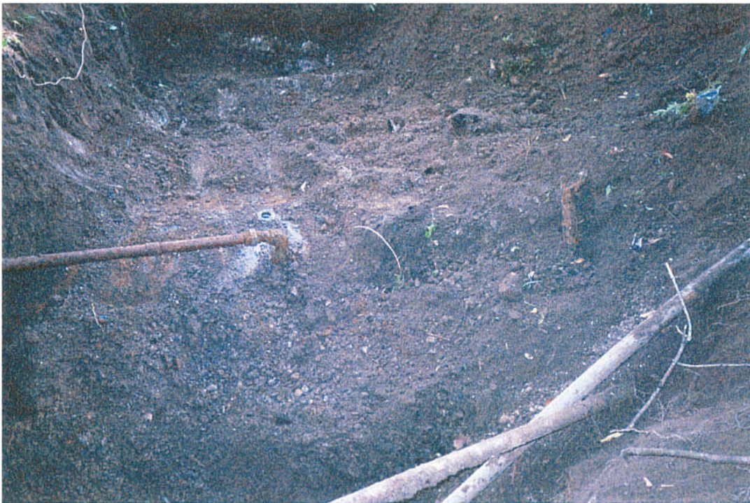
Top: Removing first UST from ground Bottom: Uncovering second UST
