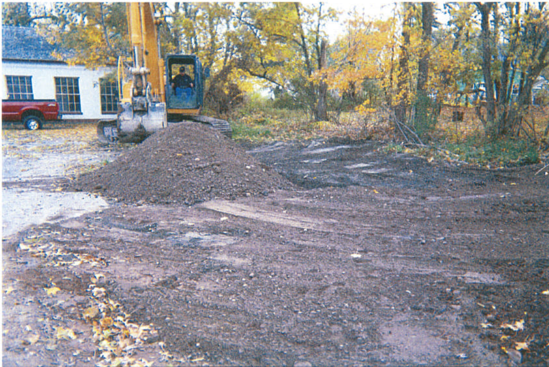
Top: Removal of groundwater from soils excavation
