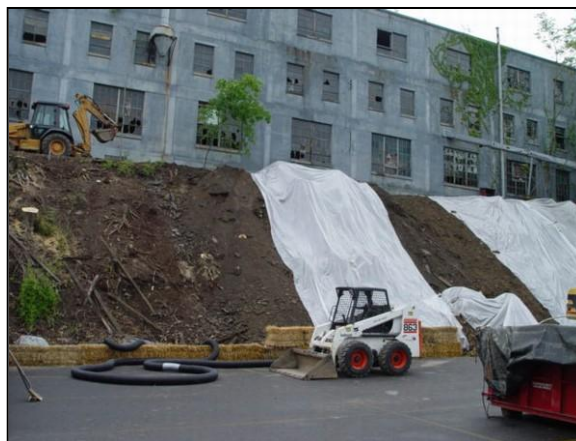
EPA remediation of portions of the Western Accessway, facing the former factory building
