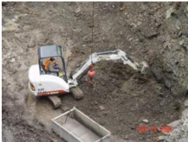
Left: EPA remediation of Plunge Pool.
