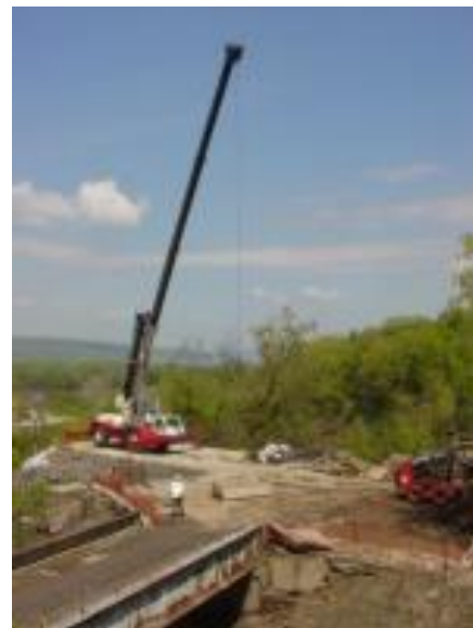
Right: EPA Remediation of Plunge Pool, Island Western Slope and Raceway. A crane was utilized to lower equipment off the island into the lower portions of the site. The crane is positioned on the former Metal Building concrete pad.
