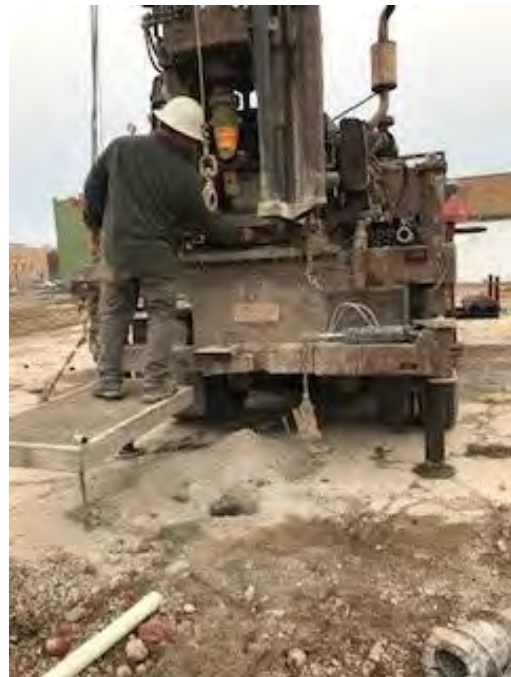
Photo No. 8 Placement of grout at MW-23
