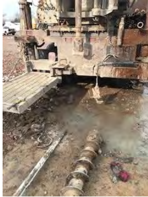
Photo No. 6 Pulled casing for MW-26 and; grouted in place
