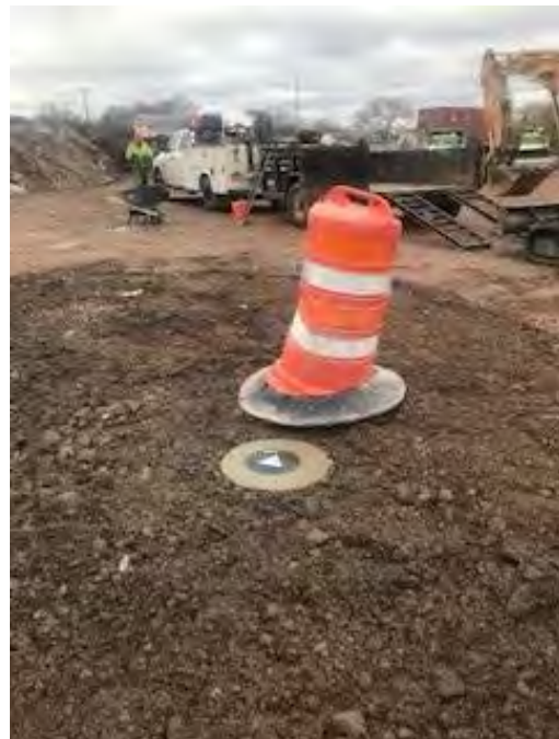
Photo No 12 MW-17 final repair
