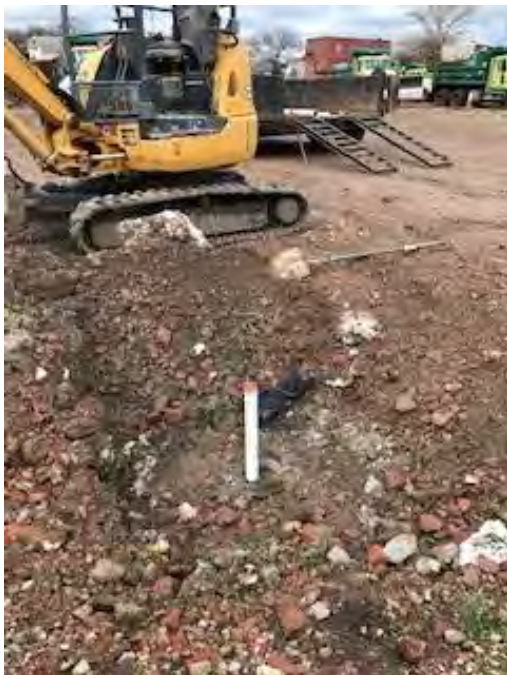
Photo No. 11 New riser implemented at MW-17
