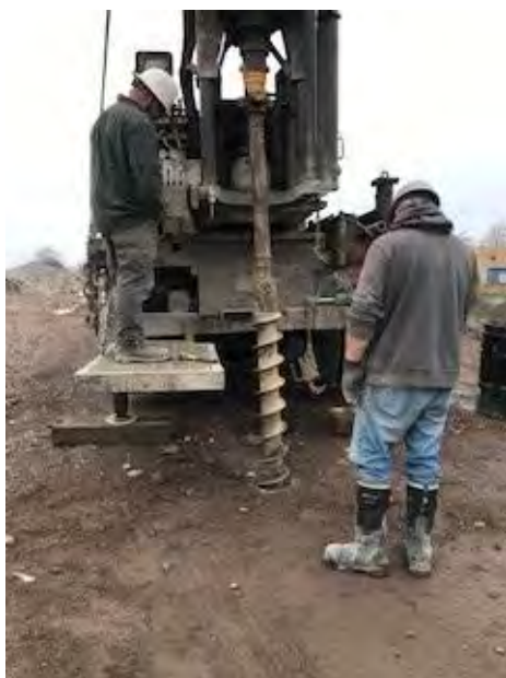
Photo No. 3 MW-22 during excavation process
