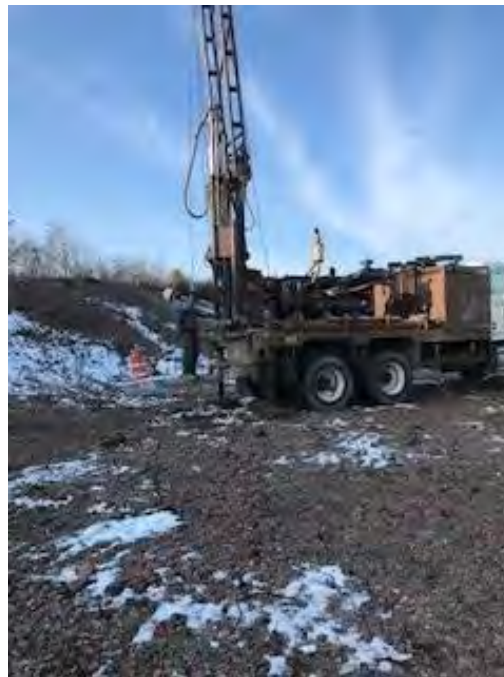
Photo No. 4 Drill rig in place at MW-29
