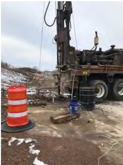
Photo No. 7 Pulling casing of MW-29
