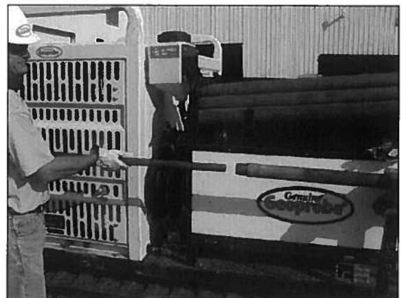
Figure 4.23. The MC5 Plug and a 1.25-inch light-weight center rod are inserted into the sample tube.
