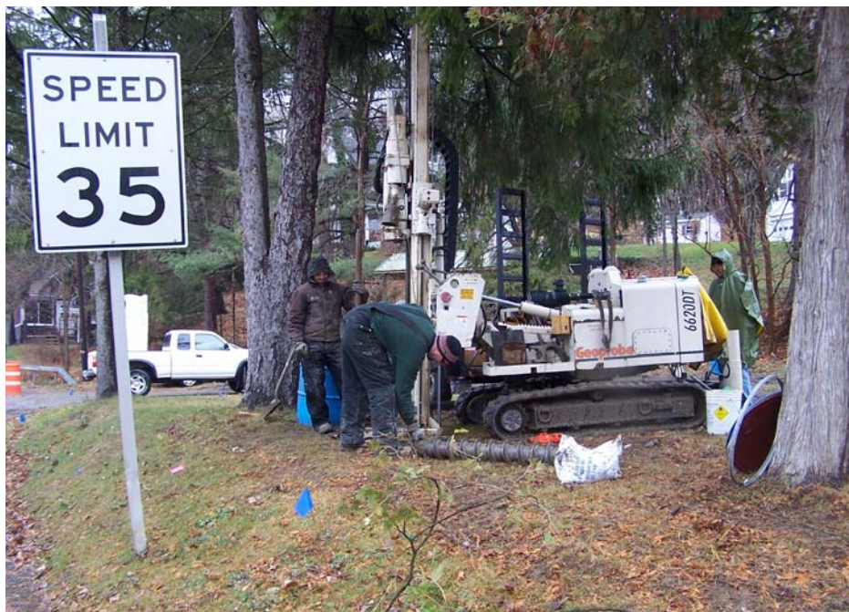
Photo No. 3. Installation of MW-6 in the right-of-way.
