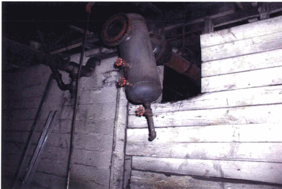
Photograph 34. Water-dispense mechanism tied to water pipes in the western portion of the structure.
