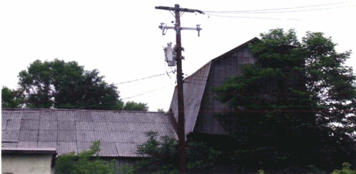
Photograph 5. Two pole mounted transformers in the southern portion of the property.
