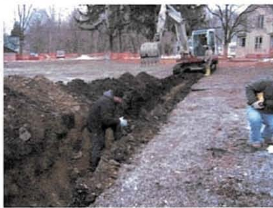
During Remediation: Excavating test trenches during the remedial investigation
