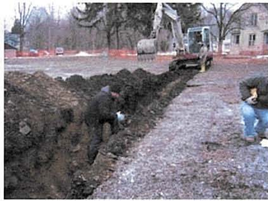
During Remediation: Excavating test trenches during the remedial investigation
