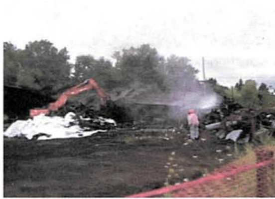
During Remediation: Implementing Interim Remedial Measure (IRM) Work Plan
