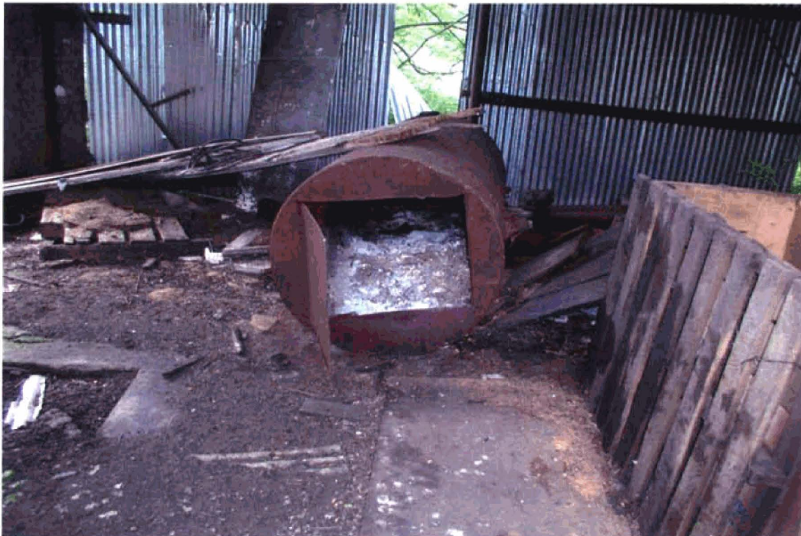
Photograph 12. Former AST used for burning of materials located in the southeastern portion of the structure.
