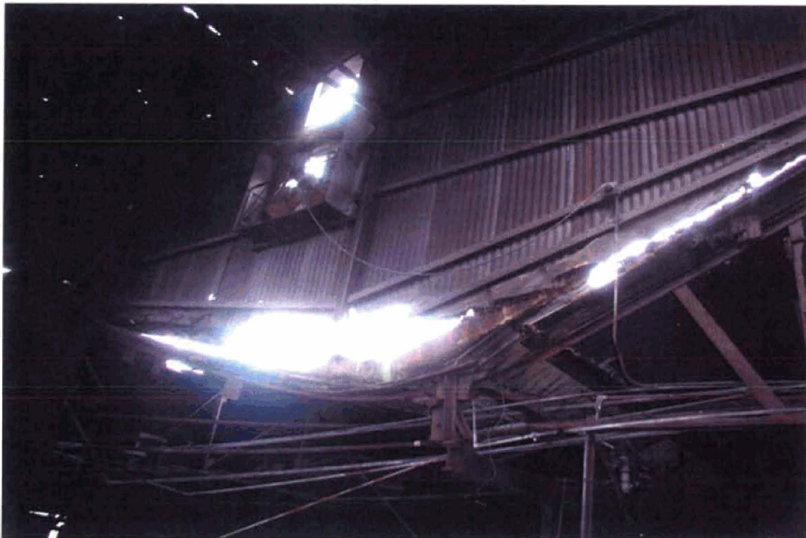
Photograph 19. Portions of ceiling and walls in the eastern area of the structure that are in disrepair.
