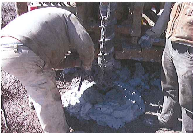
Photograph 23. Lime coming from the augers at location PEI-BH-03
