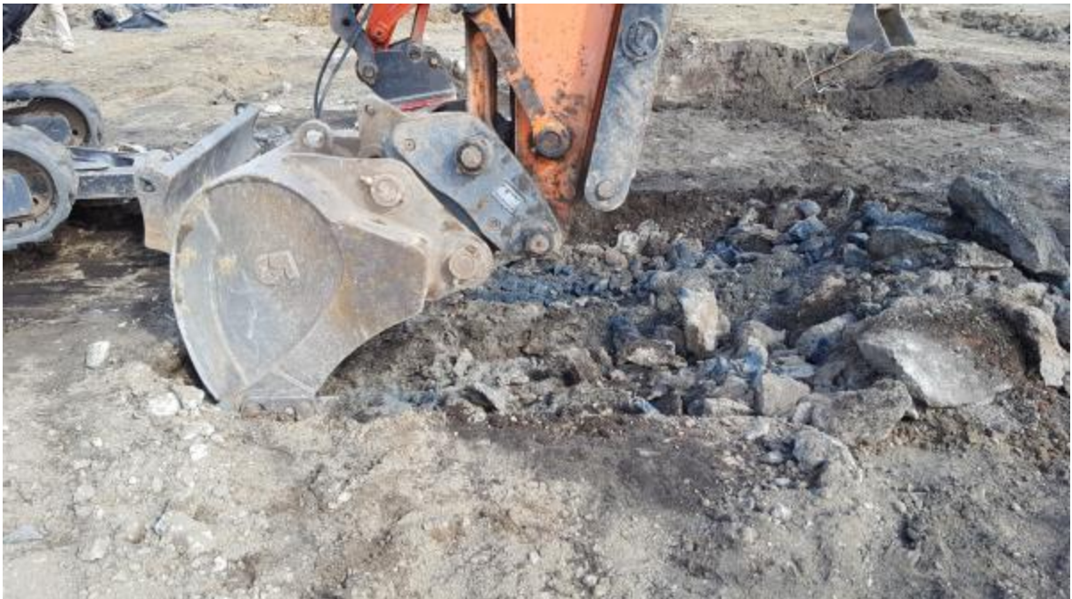
Photo 25 : Breaking out slag at westernmost pier.
