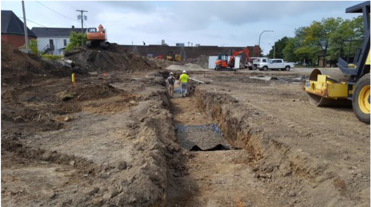
Photo 39 : View facing south from northwestern building corner.
