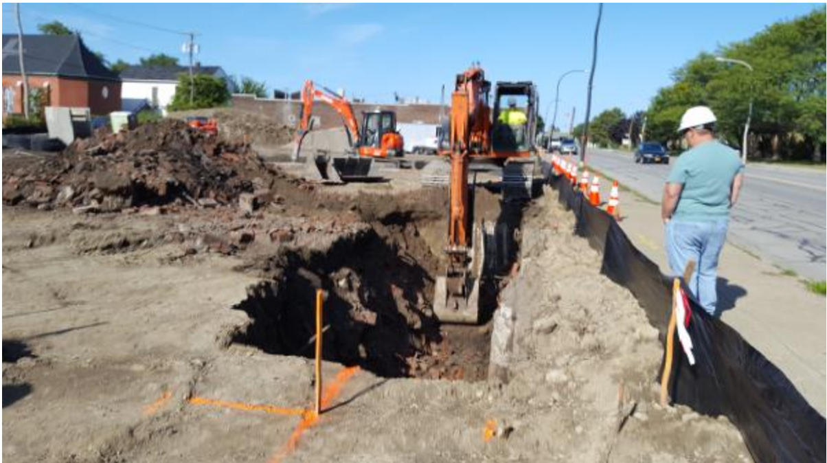
Photo 7 : Excavation for footings at northeastern corner of new building.
