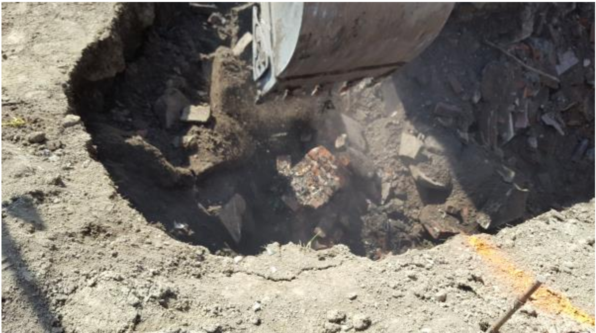
Photo 11 : Closeup of old basement floor slab thickness encountered in Area "A".
