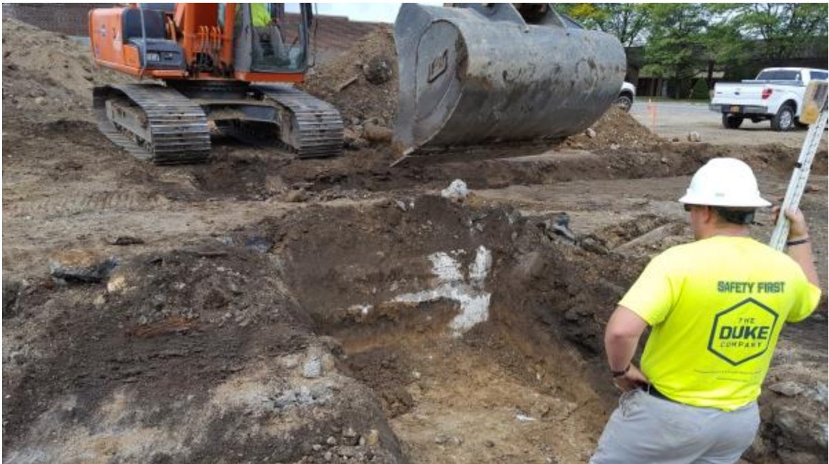
Photo 33 : Excavating for southern building footings. Minimal fills encountered in this area.
