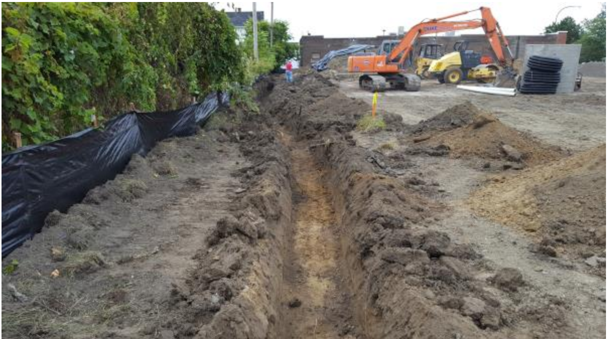
Photo 5 : Old footings and C&D fills – east of bend at southwestern corner
