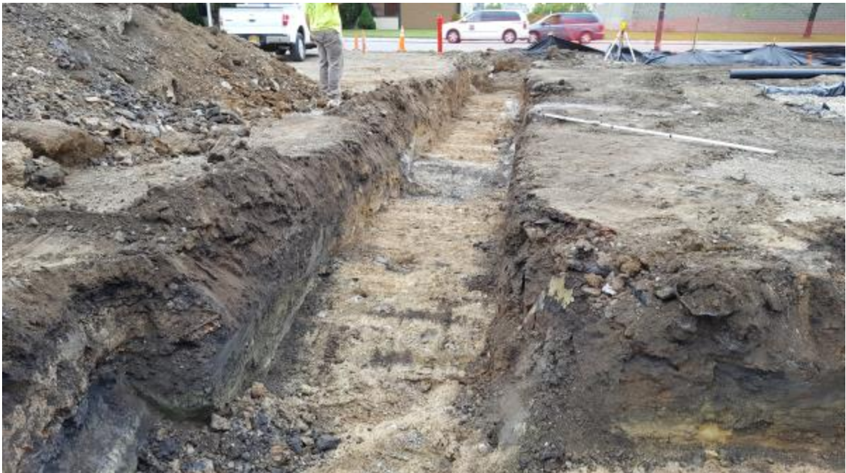
Photo 35 : View of excavation facing east from southwestern building corner.
