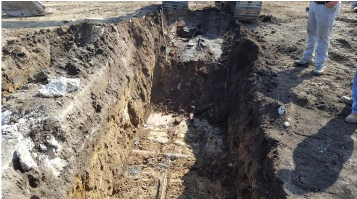
Photo 23 : Removing fills and old concrete walls at pier locations.
