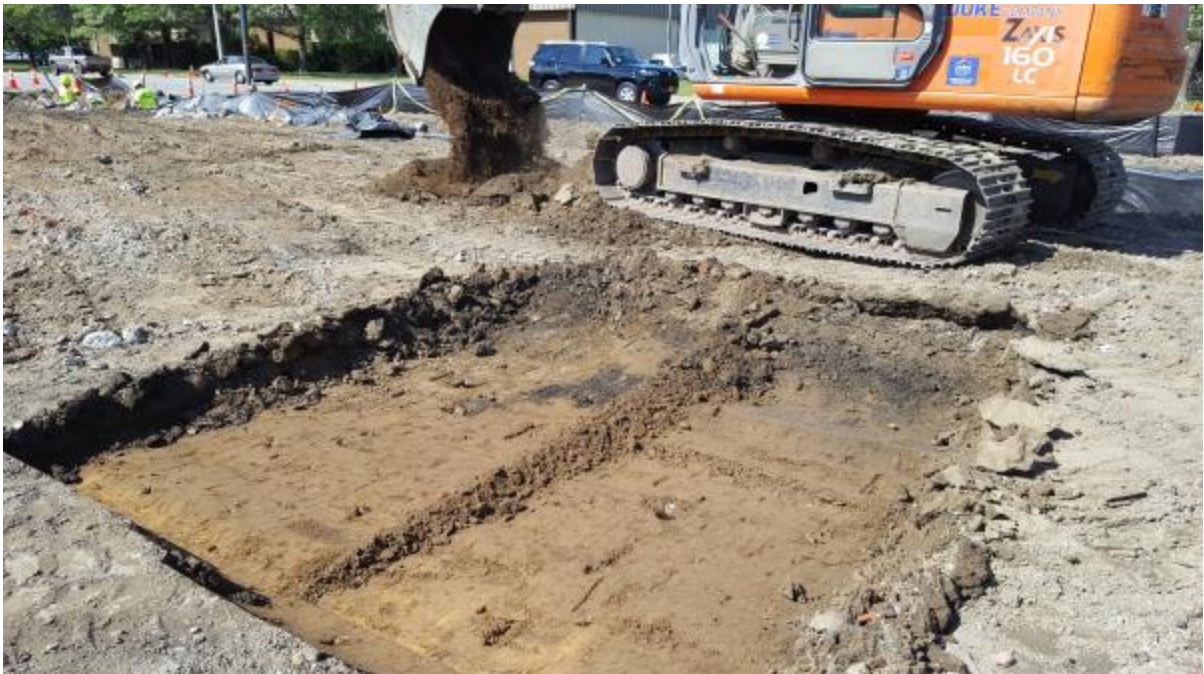
Photo 19 : Excavation of easternmost interior pier for new building.
