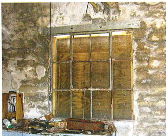
Main Warehouse – ACM Window Glazing Compound
