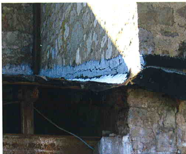
Main Warehouse – Roof Cement on Flashing
