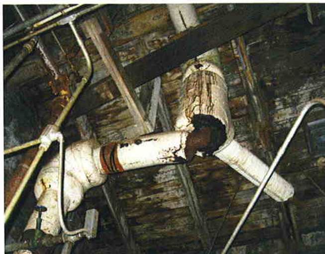
Main Warehouse – ACM Cloth Wrap on Cork Insulation
