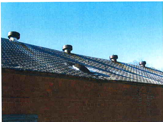
Ice House - ACM Roofing Material
