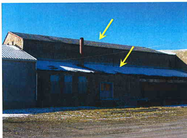
Main Warehouse – Two layers of Roof Material on Roofs
