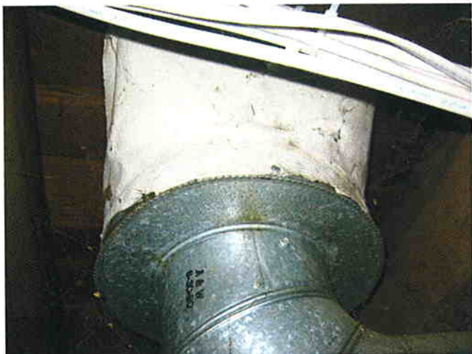
House- Cloth Wrap on Ductwork in Basement
