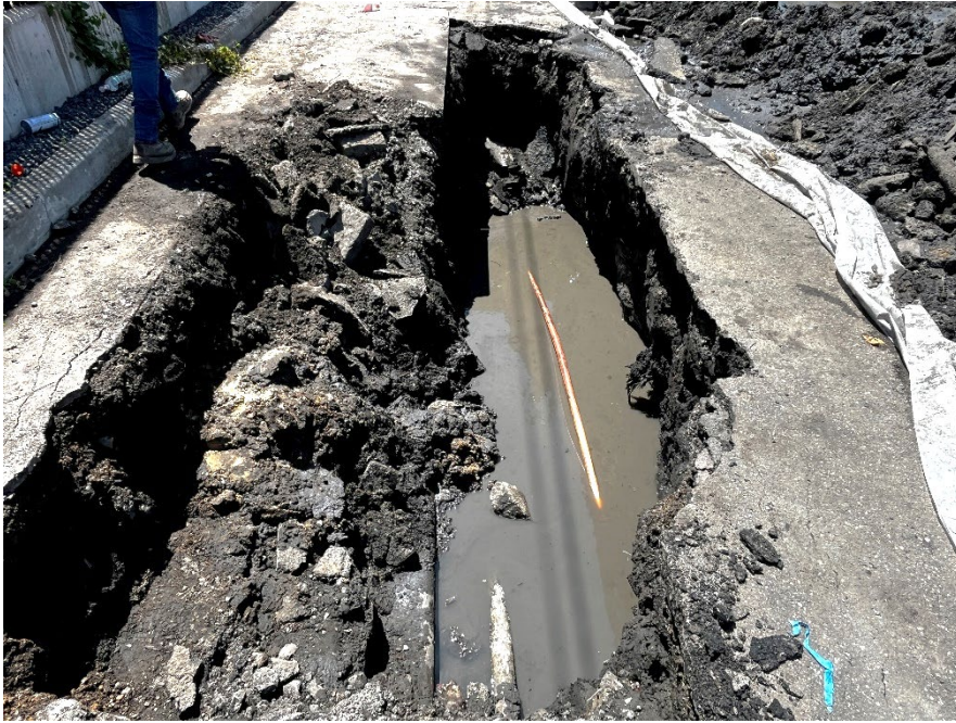
Photo 3: New copper pipe installed.
