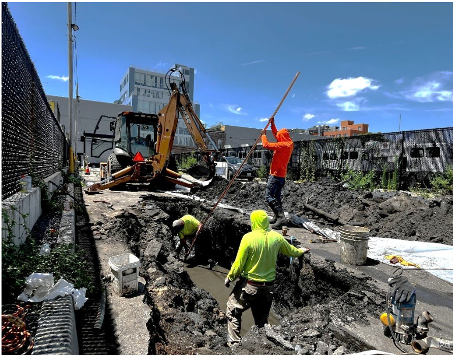
Photo 2: Smiley Waterworks replacing the broken water pipe with a new 2" copper pipe.
