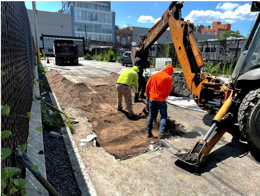
Photo 4: Smiley Waterworks tamping and grading backfill delivered from Allocco Recycling Ltd.
