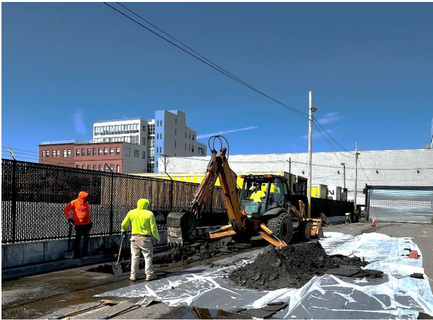
Photo 1: Smiley Waterworks excavating to expose the broken water pipe. Stockpiling excavated soil on poly sheeting.
