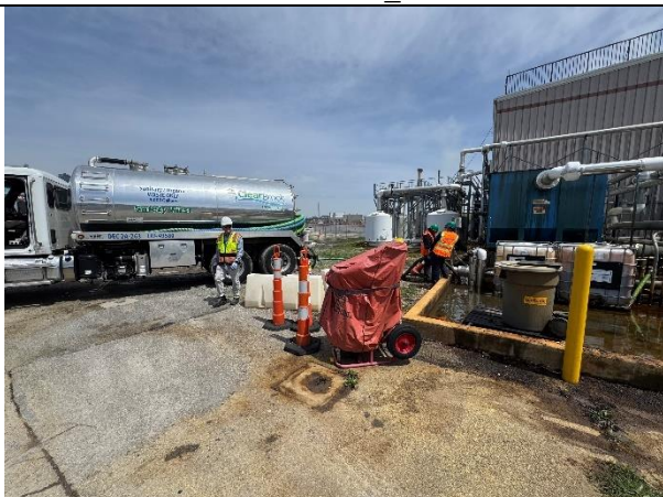
ClearBrook pumping water out of the frac tank secondary containment. 042525 - IMG_1858
