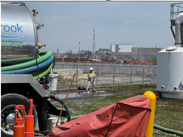
Sorbent pads being deployed to remove sheen from surface water. 042525 - IMG_1859
