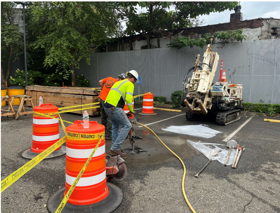
Photo 2: View facing south. View of ADT removing concrete and asphalt with a jackhammer.
