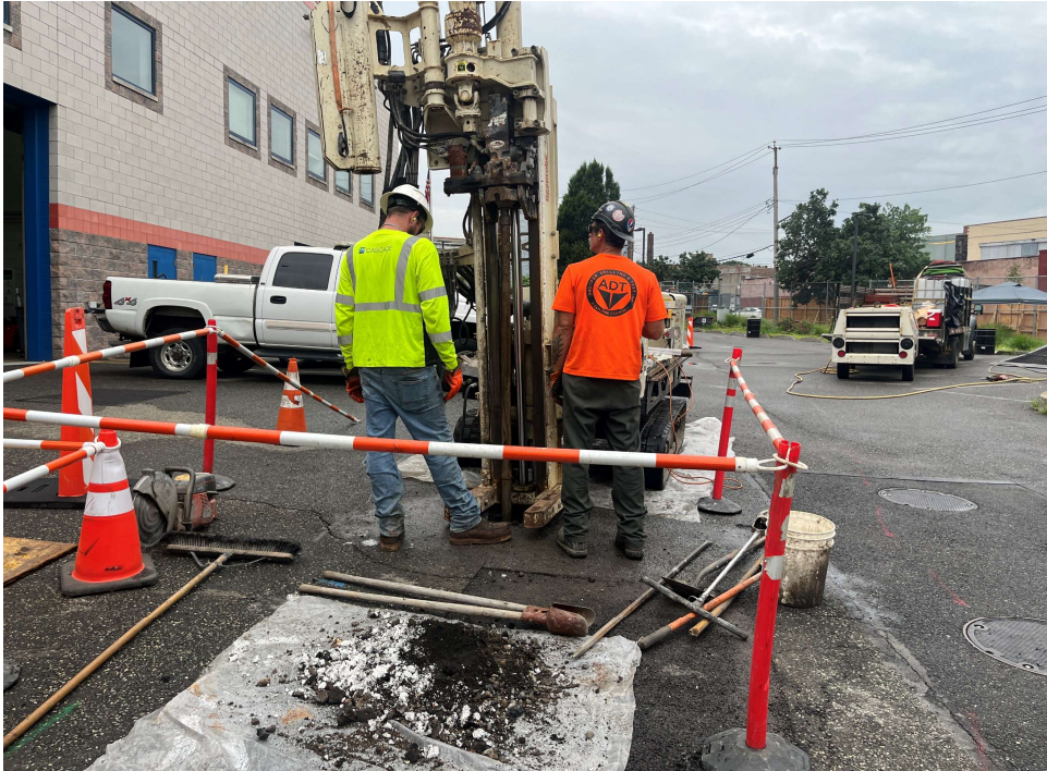
Photo 1: View facing south. View of ADT drilling to 8 ft bls.
