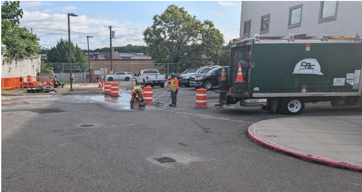
Photo 2: View facing north. View of CAC saw cutting asphalt.
