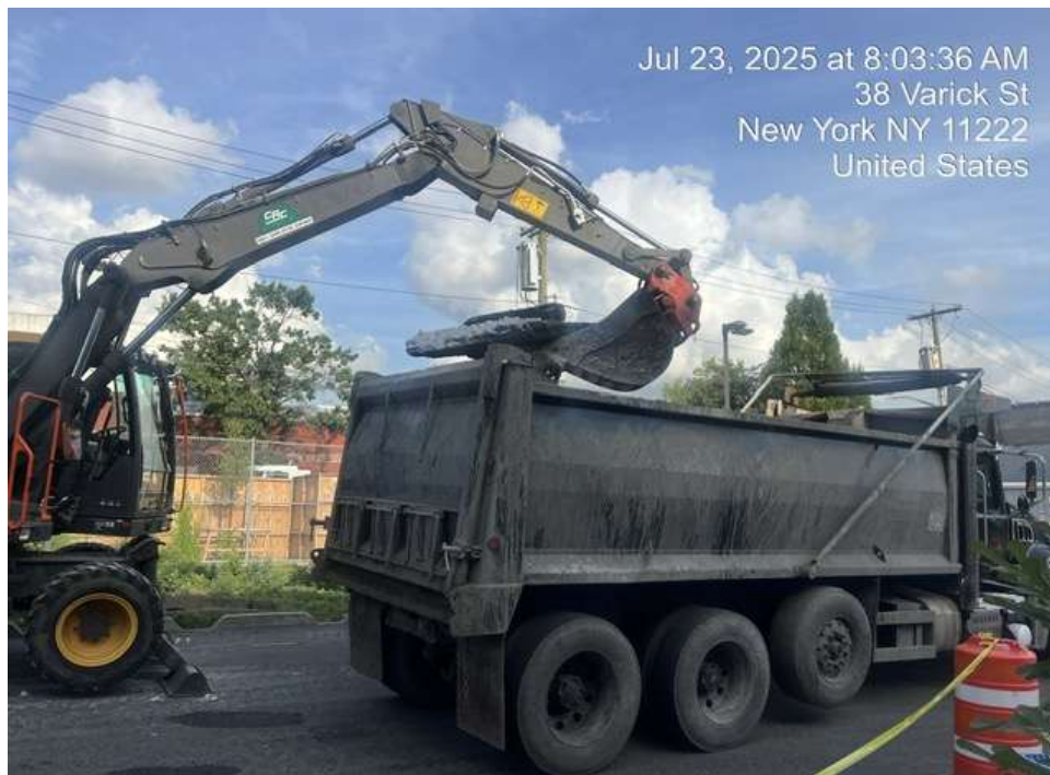
Photo 2: View facing west. View of Contractor removing asphalt driveway.
