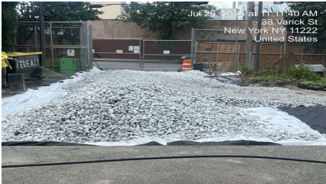
Photo 1: View facing Southwest; worker spraying water for dust suppression for newly installed construction entrance
