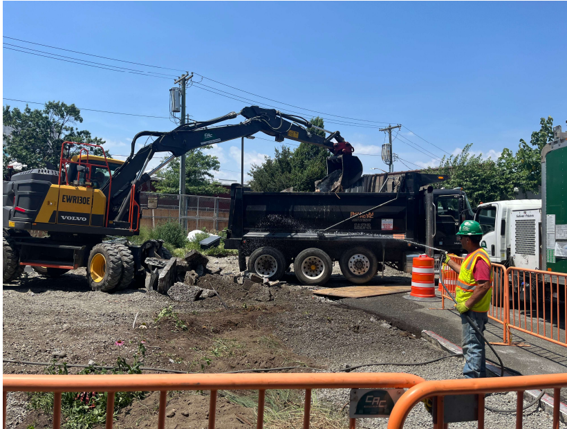
Photo 1: View facing southwest. Worker spraying water for dust suppression for concrete being removed from site.
