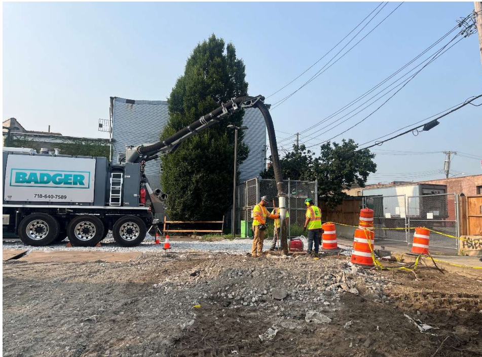
Photo 1: View facing south. CAC using guzzler vacuum truck to soft dig for utility trenches for RW-I utility relocation.
