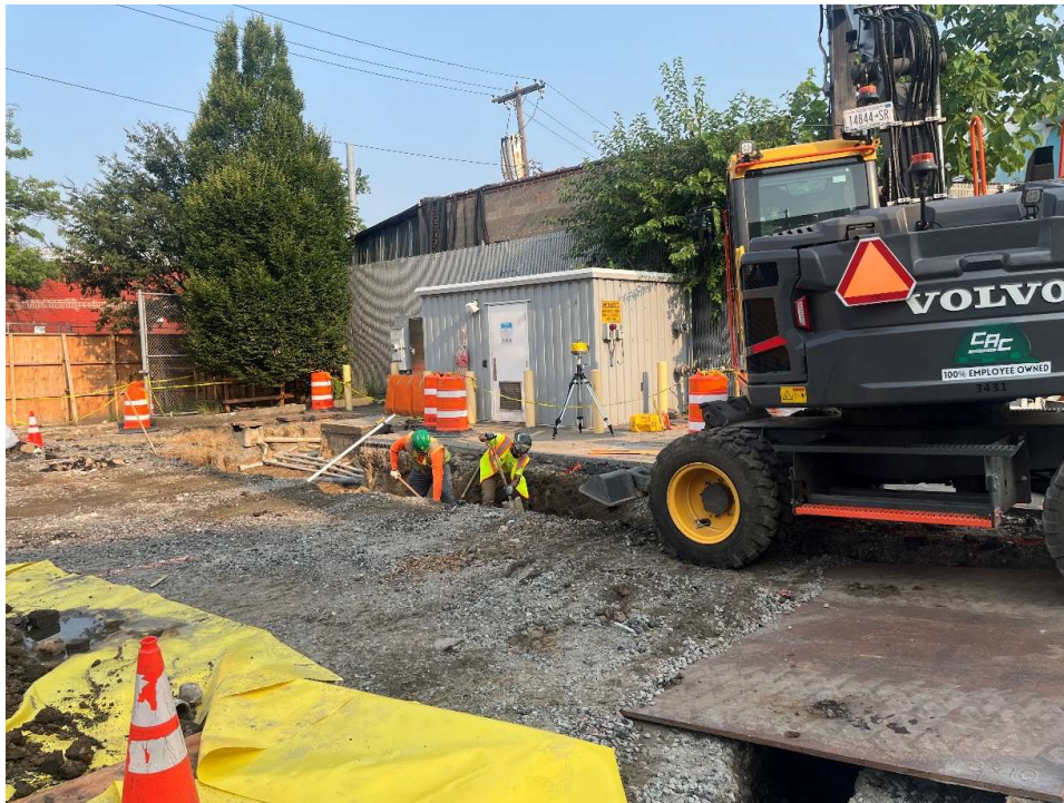
Photo 2: View facing north. CAC digging trench for utility installation including RW-I modification.
