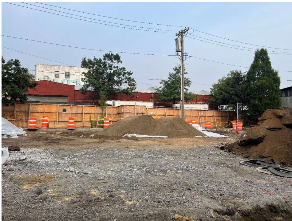
Photo 2: View facing west. View of imported concrete sand stockpiled on poly sheeting.
