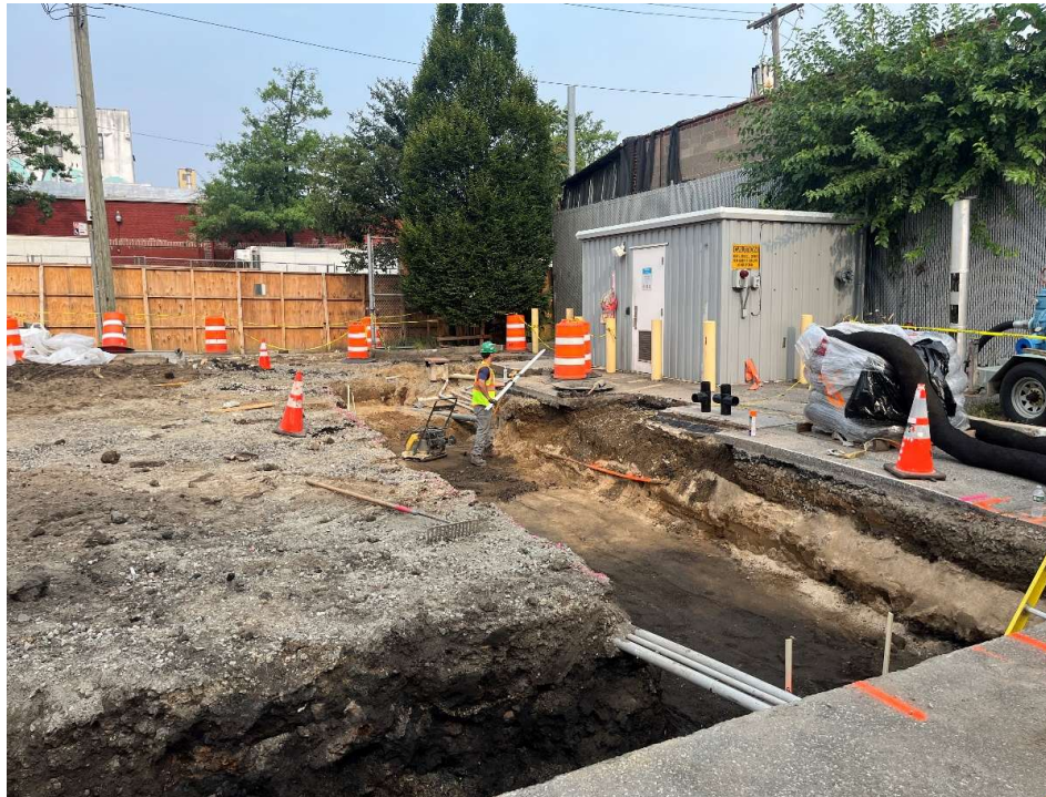
Photo 1: View facing northwest. CAC expanding the trench for RW-I modifications and relocation of associated piping.
