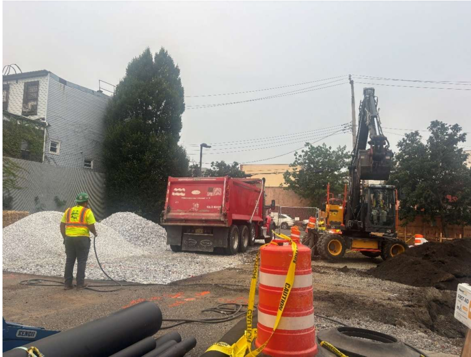
Photo 1: View facing west. CAC loading a truck with material for Clean Earth, and CAC performing dust suppression with water.
