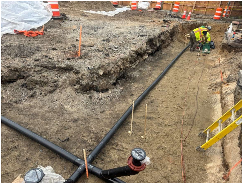
Photo 2: View facing west. View of CAC installing piping in the trench on top of compacted concrete sand.
