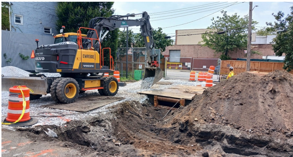
Photo 2: View facing south-southwest. View of CAC after placement of the trench box and plates.
