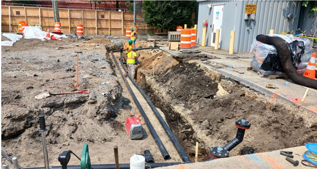
Photo 1: View facing northwest. CAC hand digging for the water service/sprinkler line.
