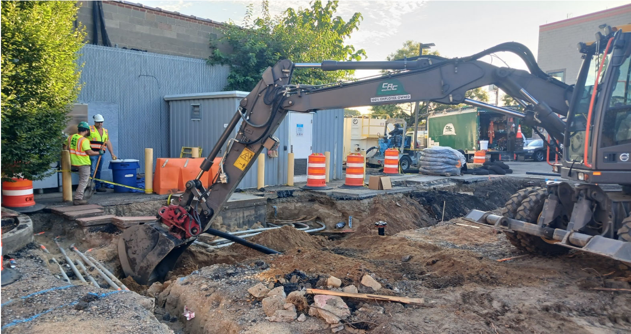
Photo 1: View facing south. View of CAC excavating and expanding the trench for RW-I modifications and relocation of associated piping.
