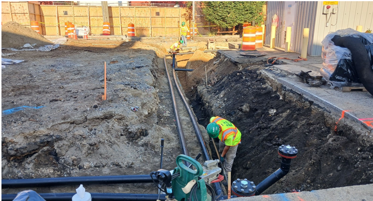
Photo 2: View facing west. View of CAC installing piping for the water/sprinkler line.
