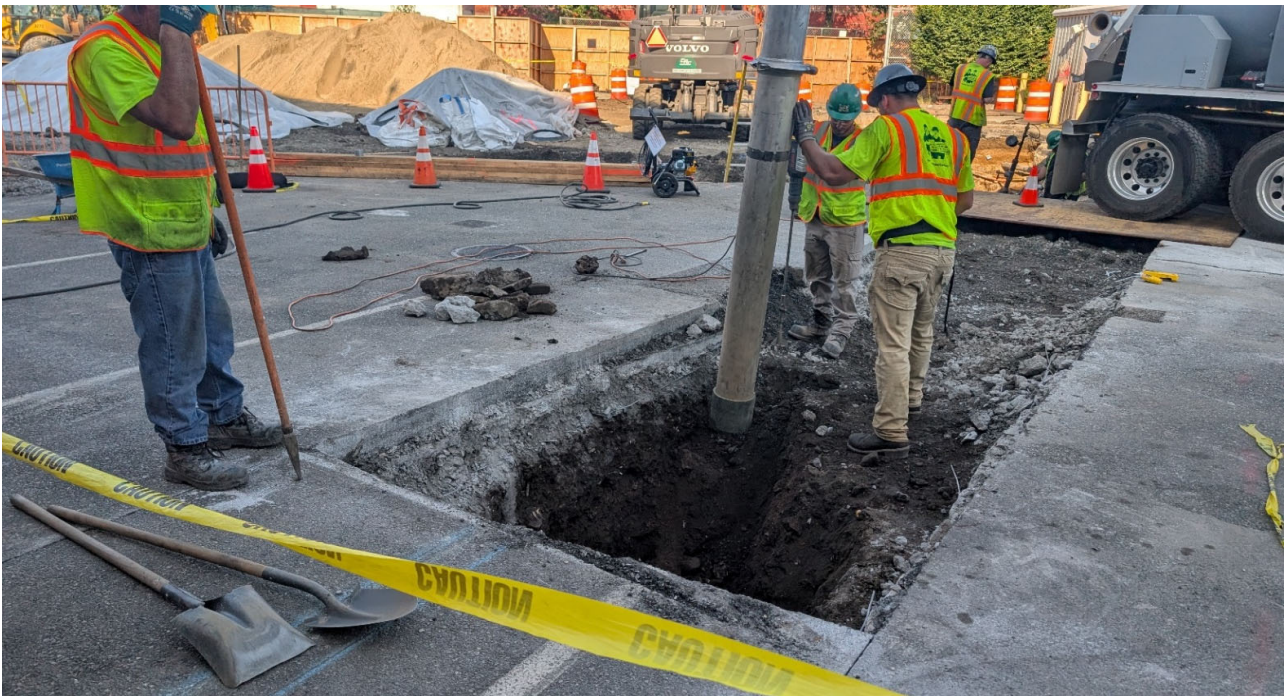
Photo 2: View facing southwest. View of CAC soft digging in utility areas for utility clearance.
