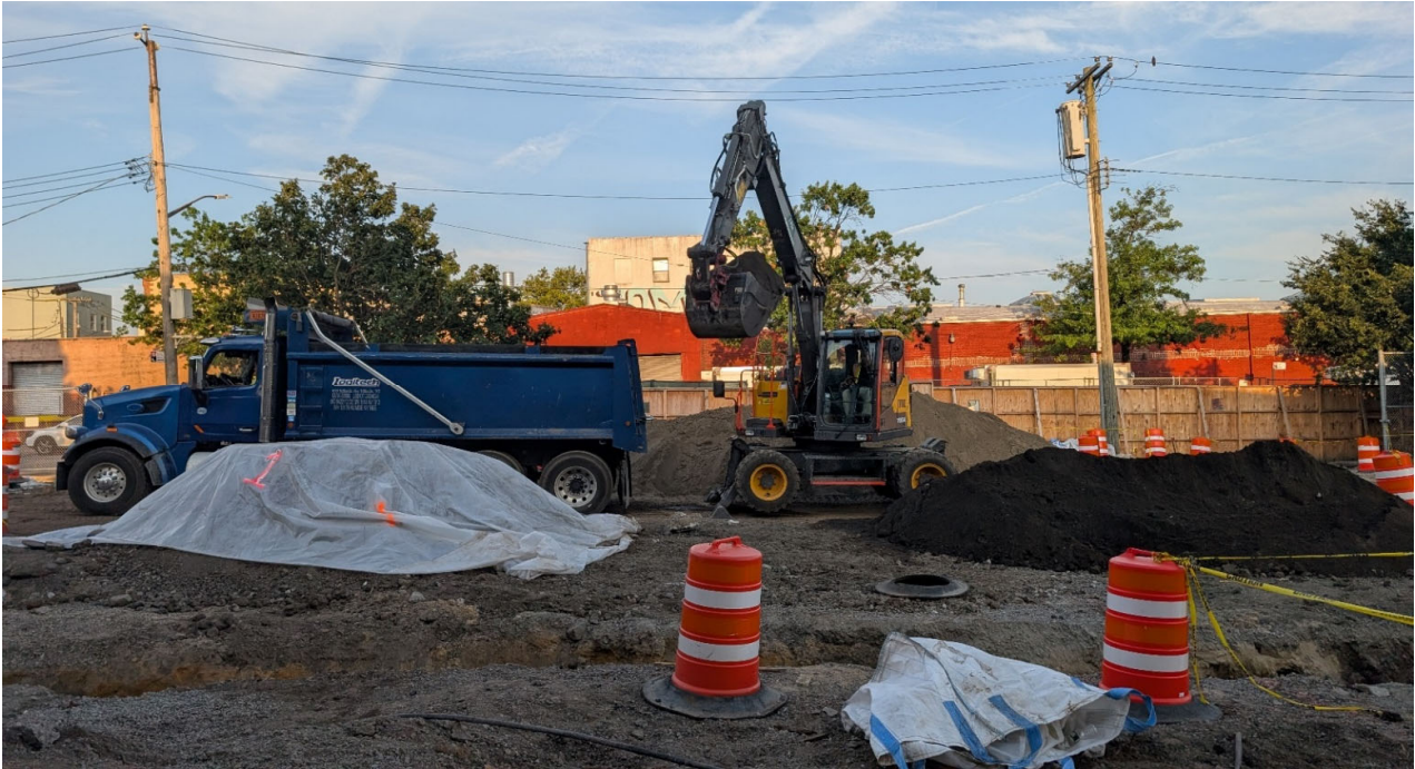
Photo 1: View facing west. View of CAC loading truck with non-hazardous soil for export.
