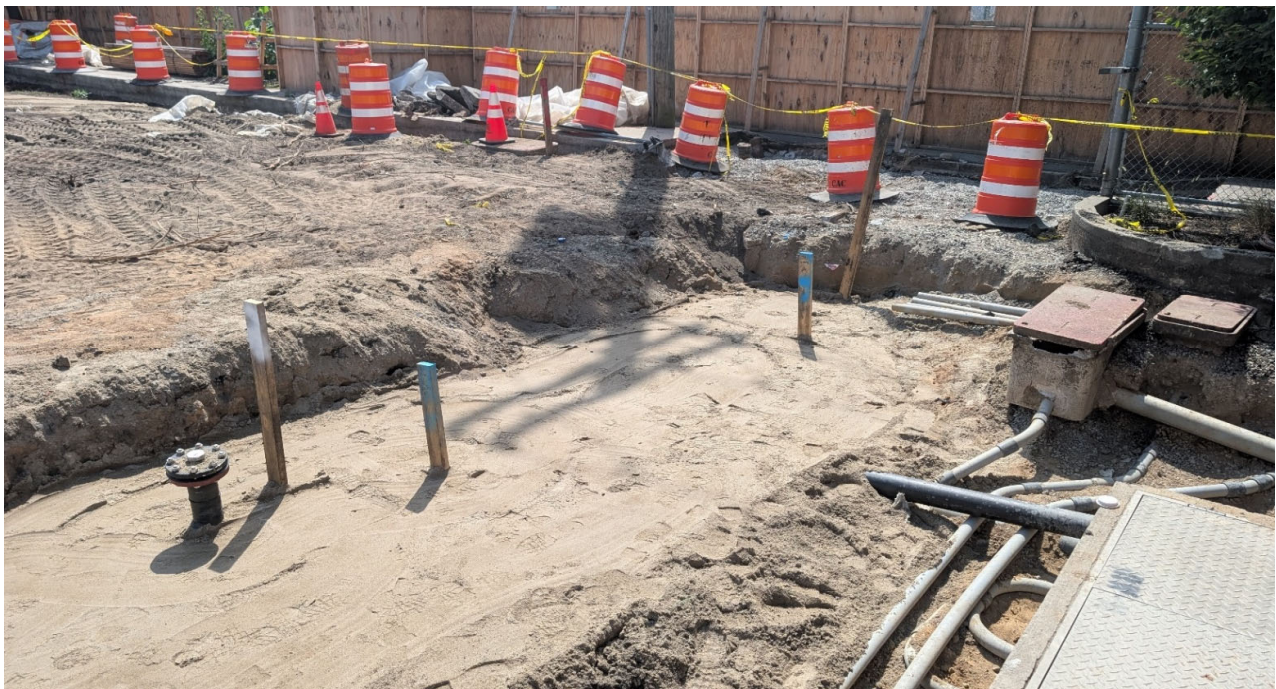
Photo 2: View facing southwest. View of trench backfilled with imported concrete sand.
