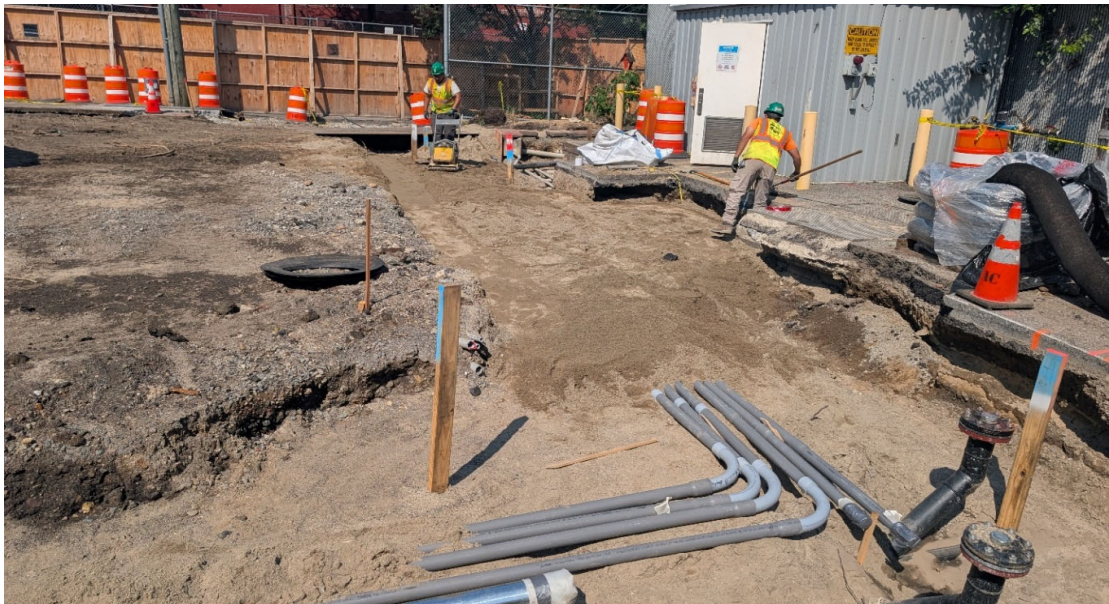
Photo 2: Backfill and compaction into electric conduit.
