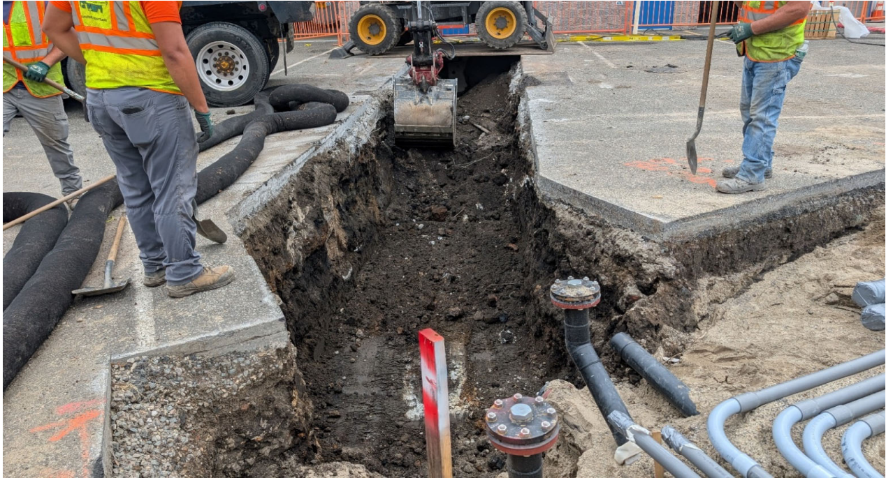
Photo 1: View facing west; View of CAC excavating soil for water trench towards new building perimeter.
