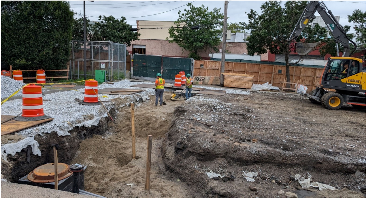
Photo 3: View facing west; View of CAC backfilling and compacting trench with imported concrete sand.
