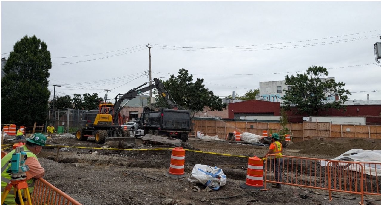
Photo 2: View facing west; View of CAC loading a truck with C&D for export and using water for dust suppression.
