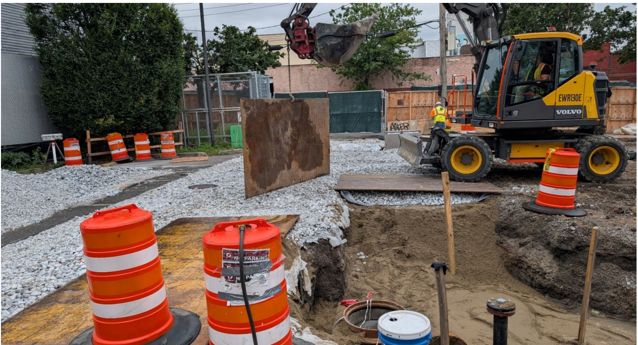
Photo 4: View facing west; View of CAC performing repairs for stabilized construction entrance.
