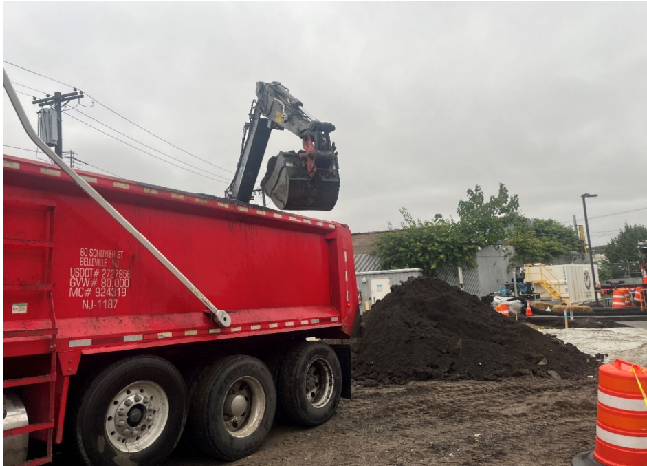
Photo 1: View facing north; View of CAC loading truck with non-hazardous soil for export.
