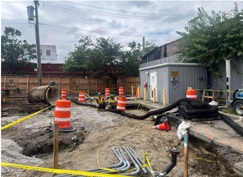
Photo 4: View facing west; View of CAC upkeep erosion and sediment controls.
