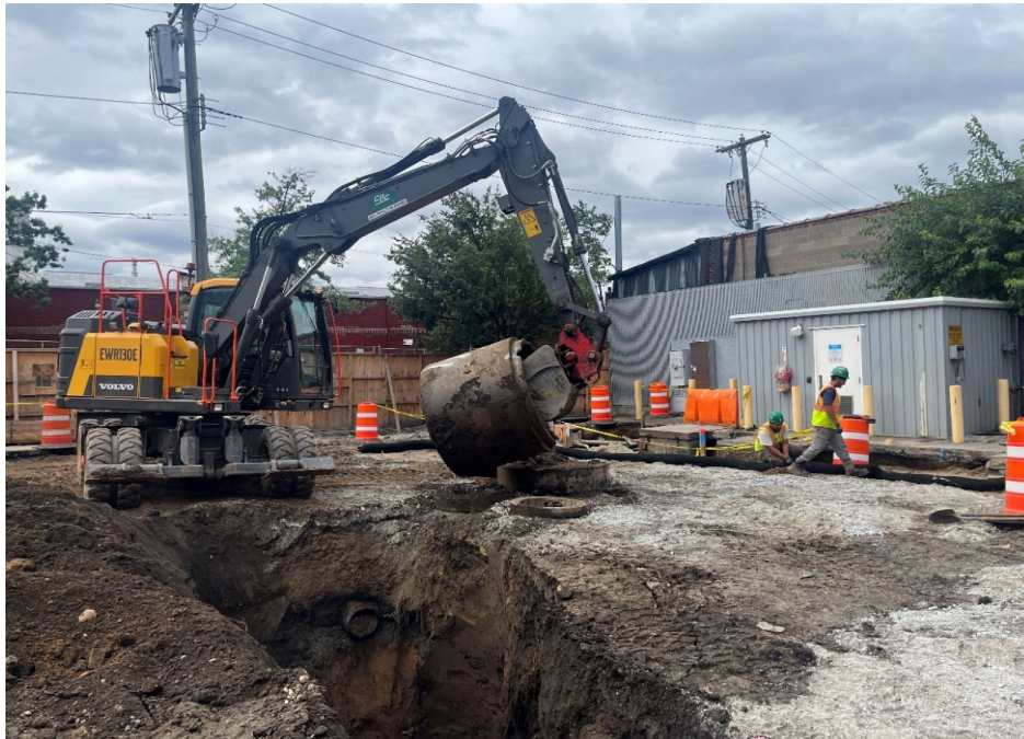
Photo 3: View facing west; View of CAC excavating manhole.
