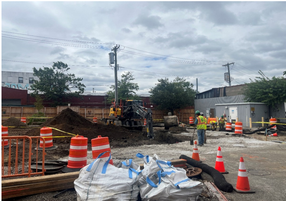
Photo 2: View facing west; View of CAC excavating soil to prepare for sheeting installation.
