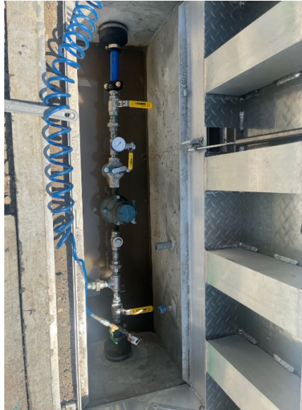
Photo 1: View facing north. Testing of secondary containment on product piping.
