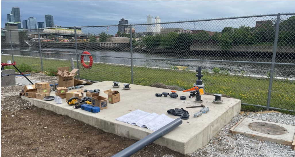
Photo 1: View facing northeast. AARCO prepping piping for upcoming assembly.
