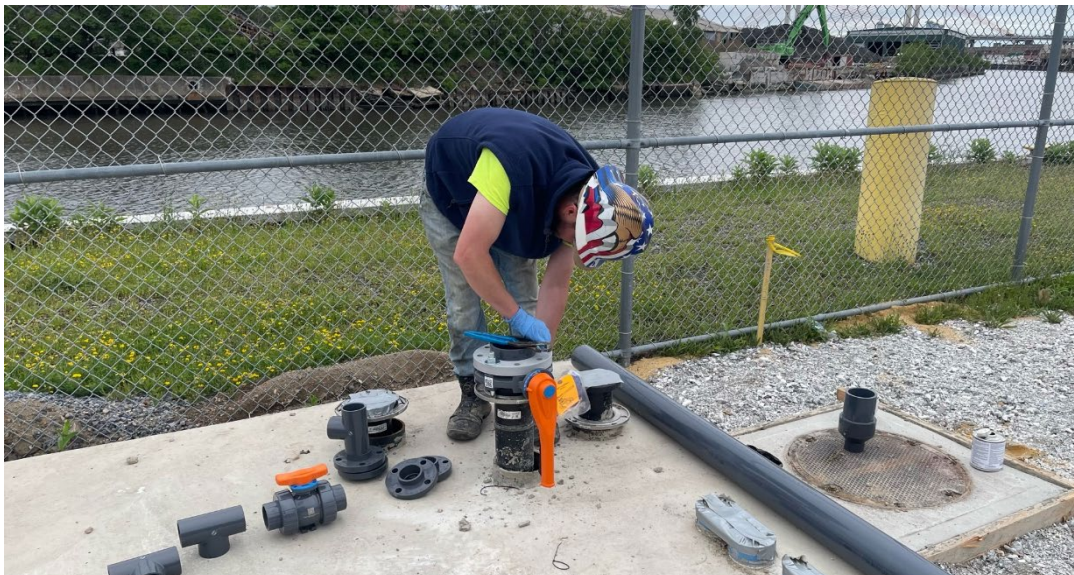
Photo 4: View facing east. View of AARCO installing piping for wellhouse.
