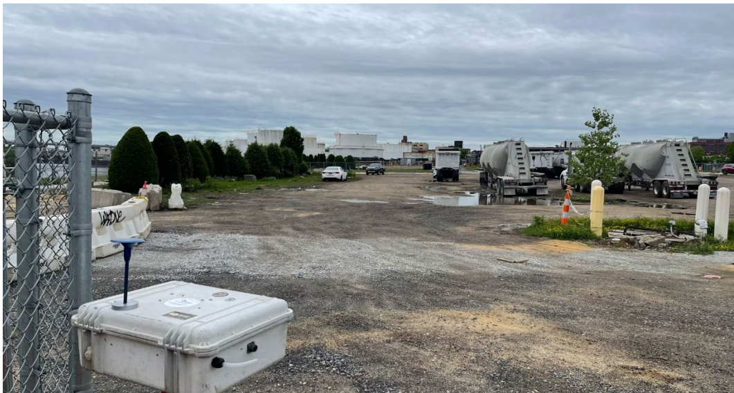
Photo 2: View facing south. View of Upwind CAMP station and general work area.
