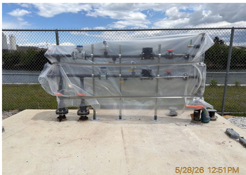
Photo 1: View facing east. Finalized piping wrapped for protection.
