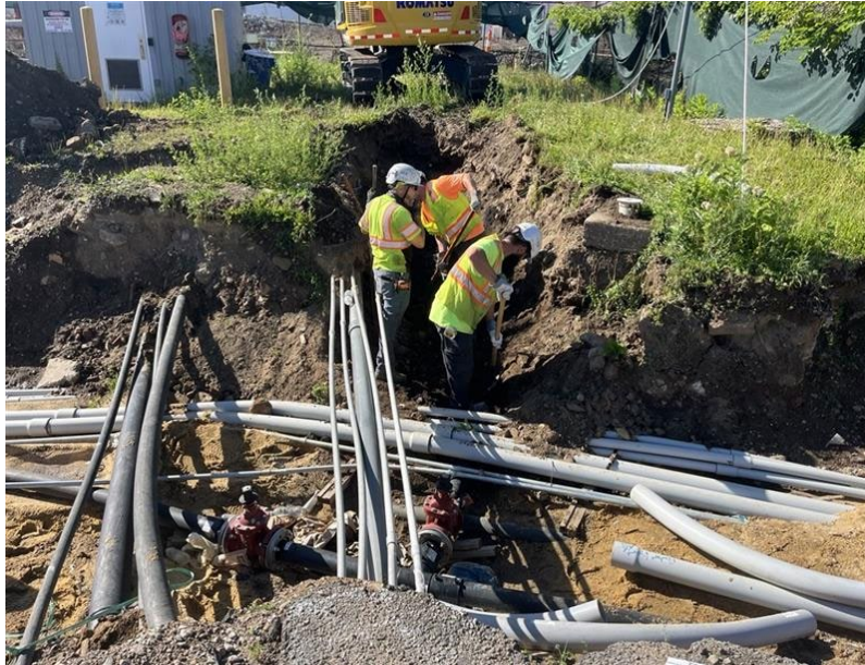
Photo 4: View facing south. View of Bancker crew soft digging in trench to exposing existing sub-surface piping.
