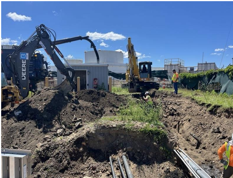
Photo 1: View facing south. Excavation of soil near Wellhouse 14.
