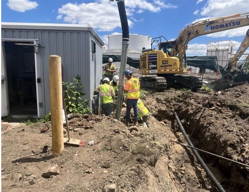
Photo 3: View facing south. View of Bancker using vacuum truck to expose existing sub-surface conduit.
