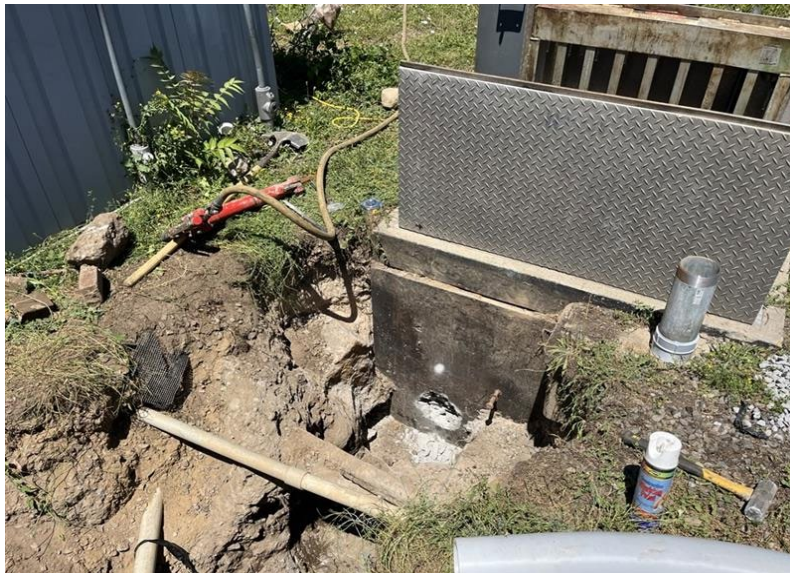
Photo 4: View facing north. View of RW-14 vault with new penetration for future new product piping.
