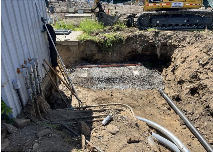
Photo 1: View facing south. View of footings for vault installation.
