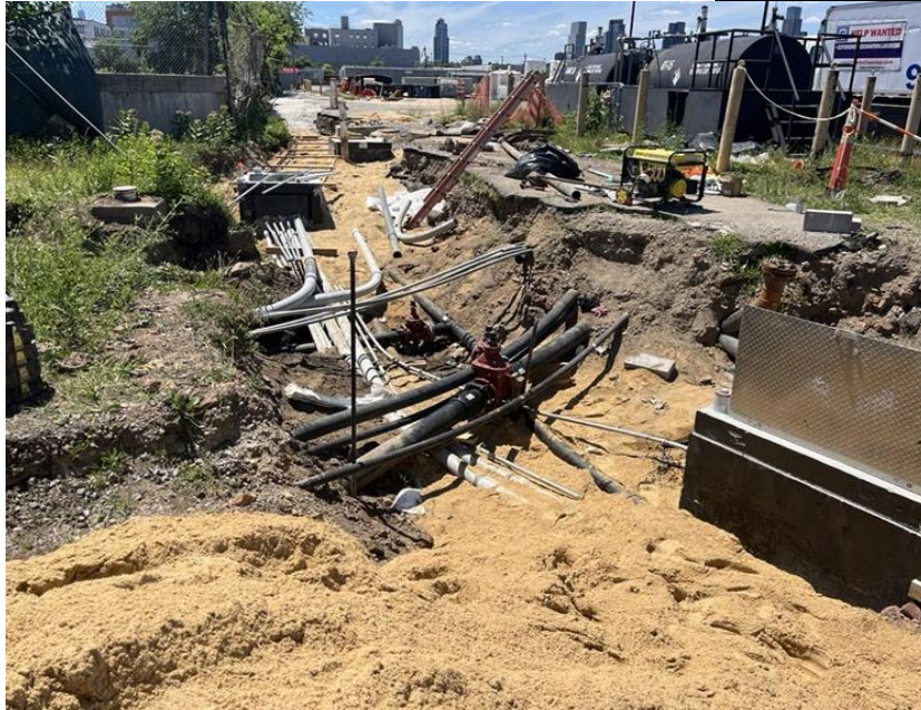
Photo 3: View facing east. View of trench along souther edge of property.
