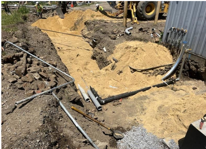
Photo 4: View facing north. View of sand being backfilled into trench over conduit near WH-14.
