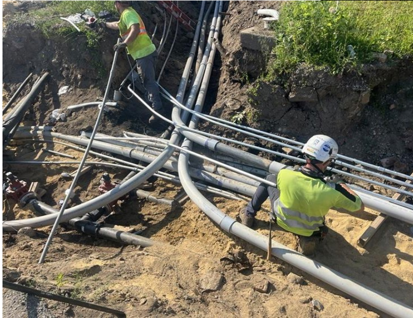
Photo 3: View facing south. View of Bancker working on fusing conduit in trench.
