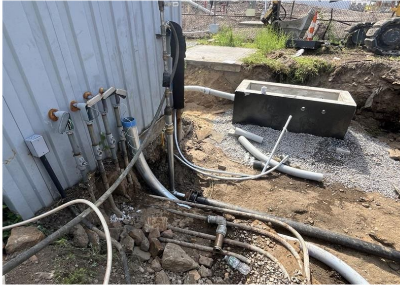
Photo 1: View facing south. View of new vault placed in trench near WH-14.
