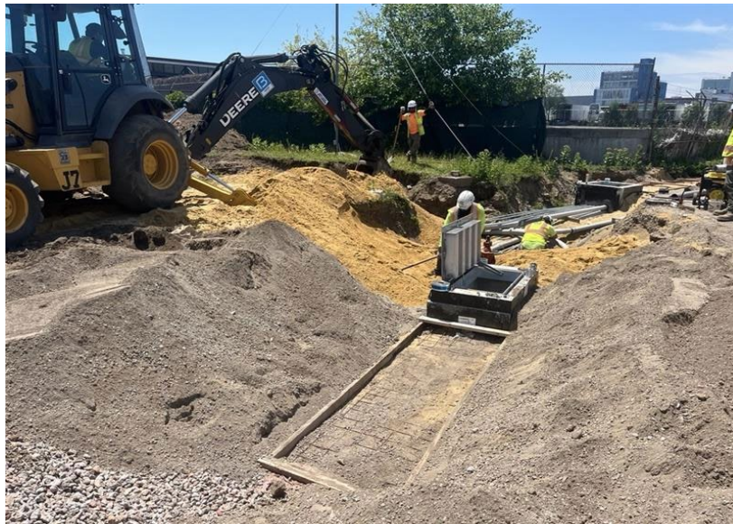
Photo 2: View facing southwest. View of Bancker setting vault at appropriate grade in trench.
