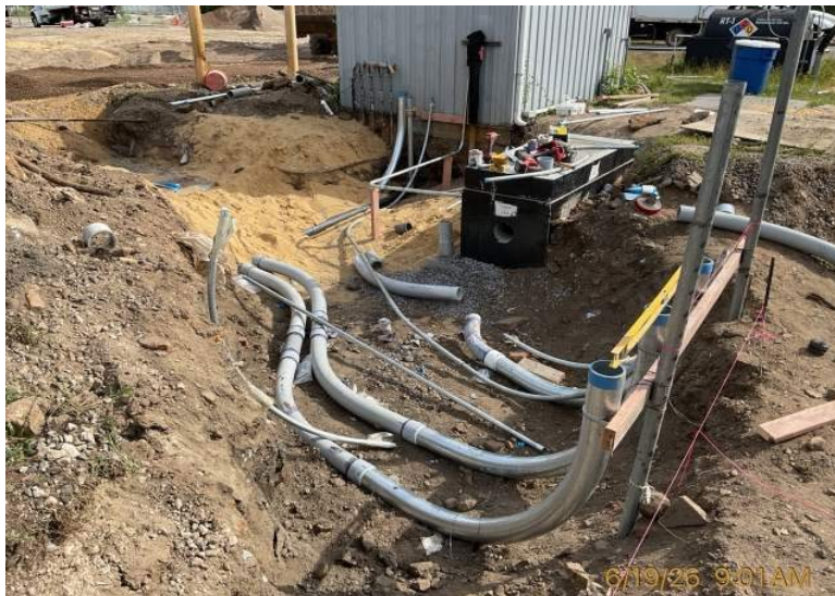
Photo 2: View facing north east. Piping installed near WH-14.
