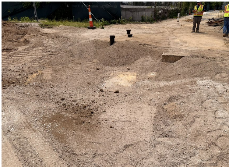
Photo 4: View facing southwest. View of backfilled trench.
