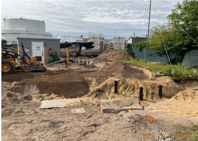
Photo 1: View facing south. Bancker backfilling trench.
