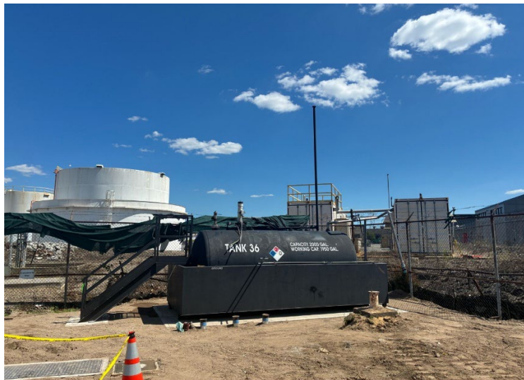
Photo 2: View facing south. New location of tank on the concrete pad.
