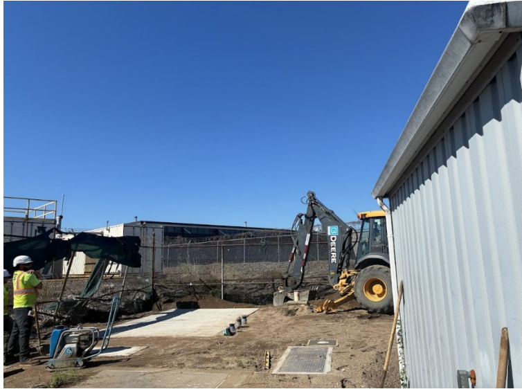
Photo 3: View facing west. Bancker continues backfilling and grading near WH-14 .
