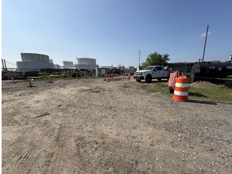
Photo 1: View facing south. View of work zone.
