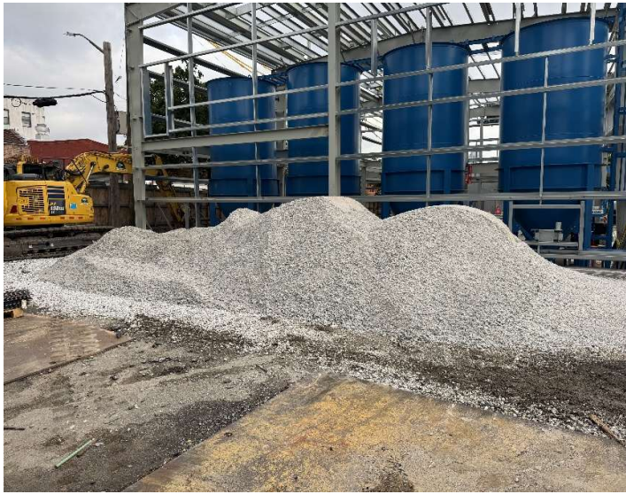
Photo 1: View facing northwest. CAC backfilling trench west of building using recent delivery of DGA stockpile.
