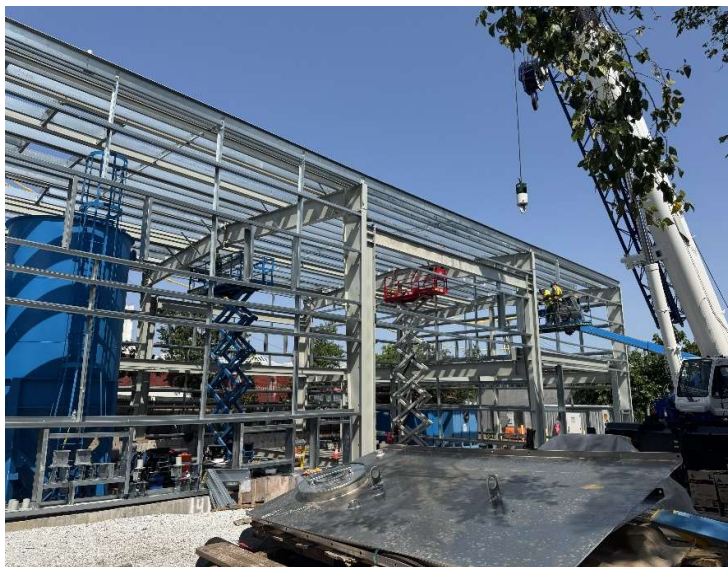
Photo 2: View facing northwest. CAC utilizing manlift and two scissor lifts to install steel building components.
