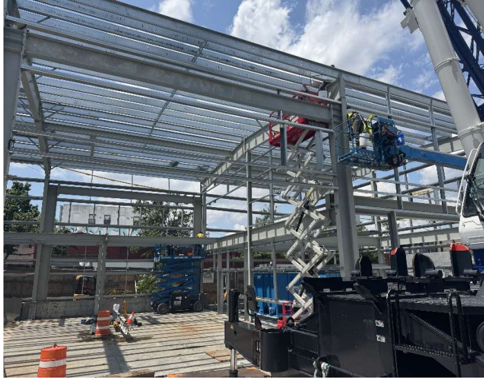
Photo 3: View facing northwest. CAC bolting up newly installed steel building components.
