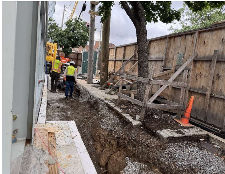
Photo 4: View facing south. CAC compacting backfilled trench west of building as CM Testing inspects the compaction.
