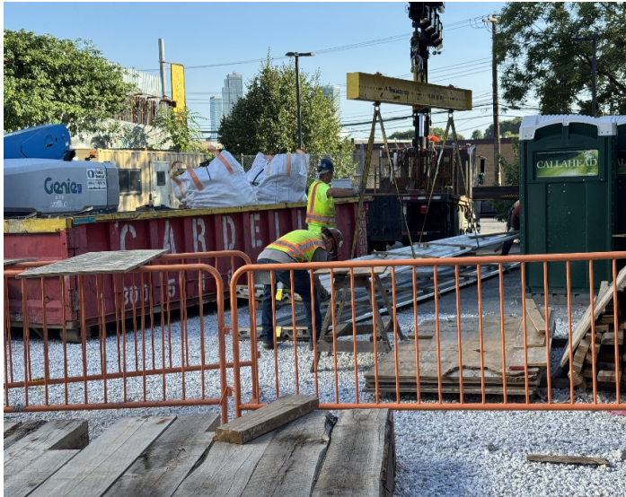
Photo 1: View facing north. CAC offloading flatbed truck with roof sheeting.
