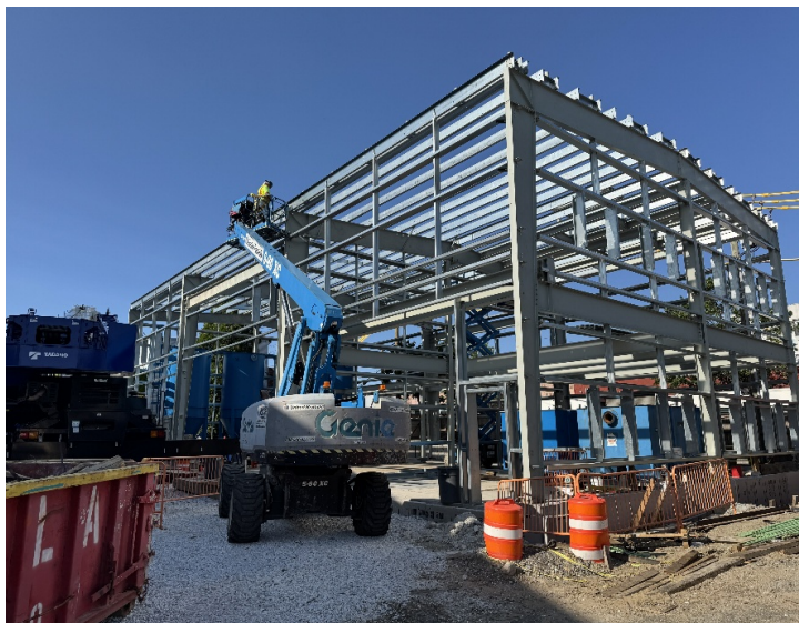
Photo 2: View facing southwest. CAC installing roof frame hardware.
