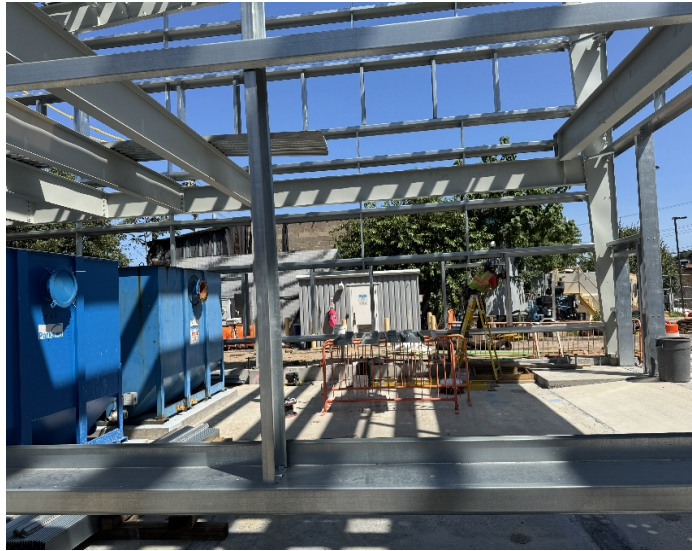
Photo 3: View facing north. CAC installing window frames on north wall of building.
