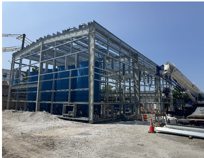
Photo 4: View facing northwest. View of steel building progress.
